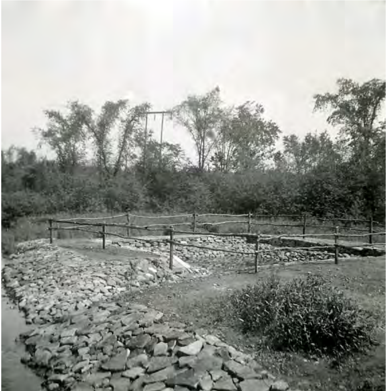
Whiskey Flats State Forest – RA 2 Proposal L, Town of Hopkinton; waterhole along Hazen Brook built in 1936. Foreman F. Strader. Remnants are still visible along the north side of State Route 72. Note the overhead powerline in the background. Waterholes were fenced to keep out livestock.
