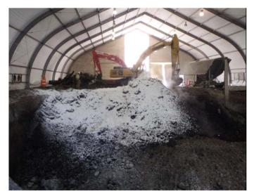
The dredged material will be loaded onto trucks in a sprung structure with an air filtration system. This controls odors, dust, and other nuisances from leaving the site.
