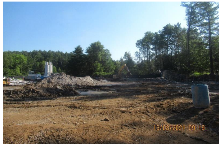
Area where ISS is complete and ready for cover material.
