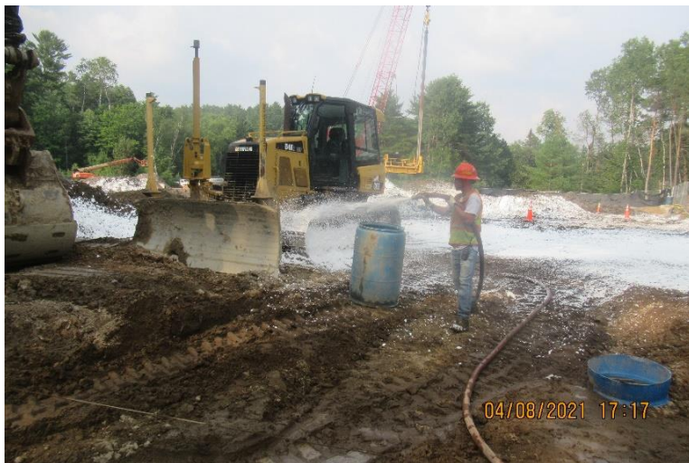
Spraying foam on exposed areas to minimize odors.
