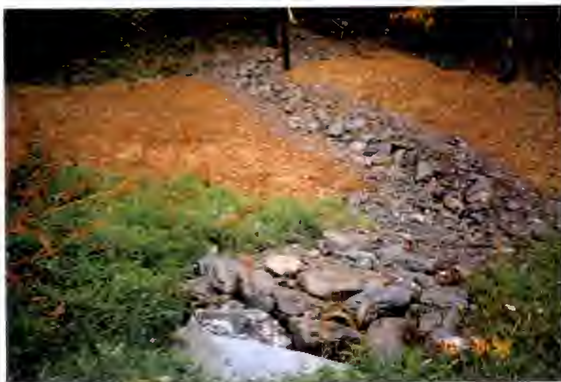
ABOVE: ESTABLISHED VEGETATIVE LAYER ON TOP SURFACE OF LANDFILL AFTER ONE SEASON OF GROWTH BELOW: RECONFIGURED DRAINAGE OUTFALL AREA AFTER INSTALLATION OF DRAINAGE BLANKET
