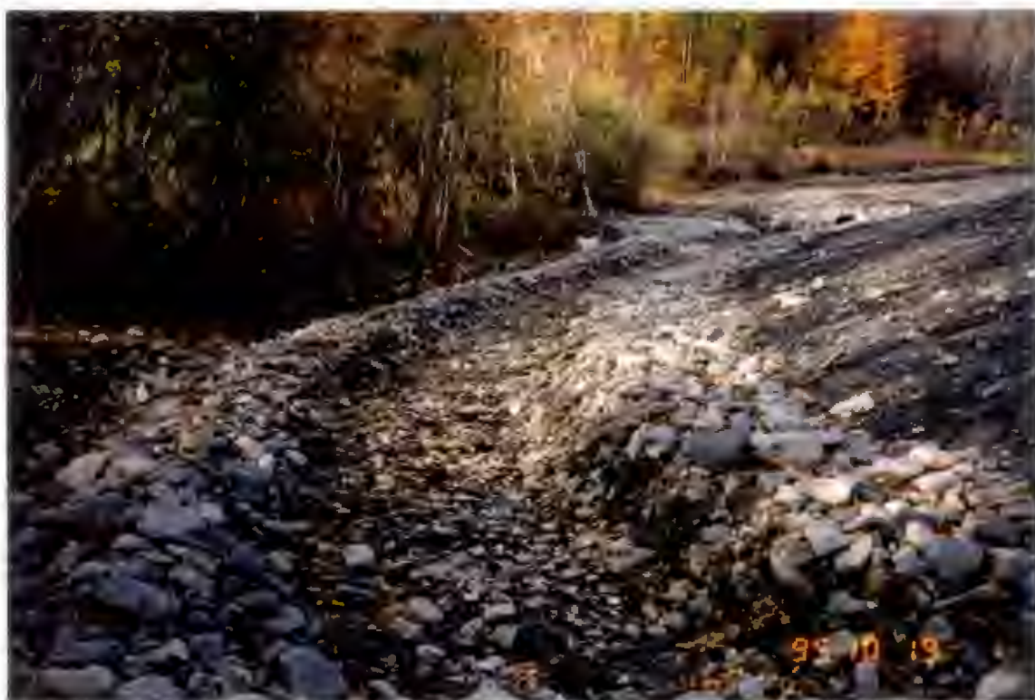
ABOVE: TOPSOIL LAYER AFTER BEING DISCED BELOW: PERIMETER TRENCH PRIOR TO INSTALLATION OF VEGETATIVE LAYER (NOTE INLET TO STREAM DIVERSION CULVERT IN UPPER RIGHT HAND CORNER)
