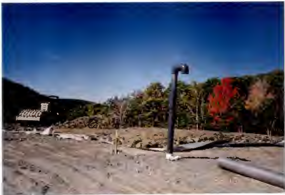
GAS VENT CONSTRUCTION
