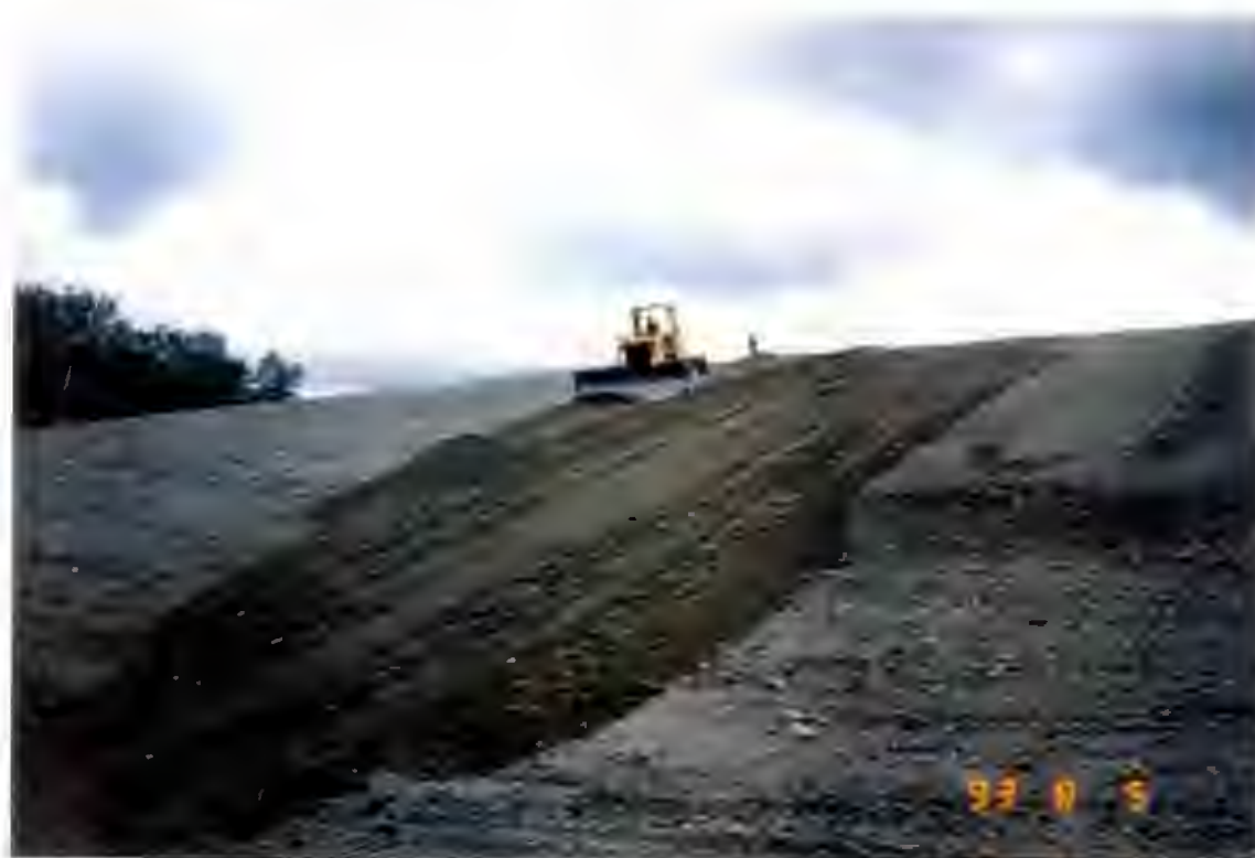
GAS VENTING SOIL LAYER PLACEMENT
