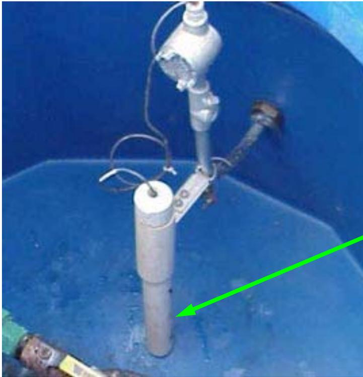
The photo at left shows a properly positioned sump sensor.
