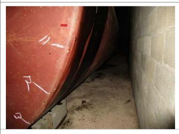
Staining Beneath #6 Fuel Oil Tanks
