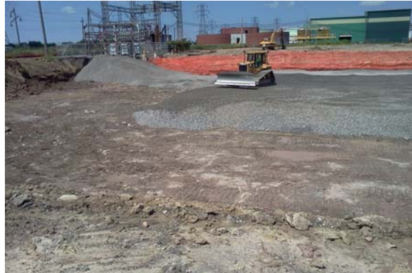
During Remediation: Site backfilling at Former Mill #2 Site
