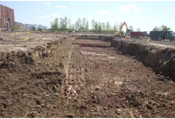
During Remediation: Soil excavation at Former Mill #2 Site
