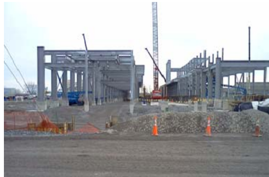
After: Former Mill #2 Site clean with redevelopment already under construction
