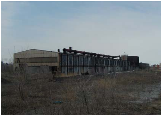
Before remediation: Northeast corner of Roblin site
