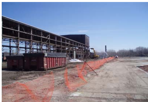
During remediation: Southwest side of building during demolition
