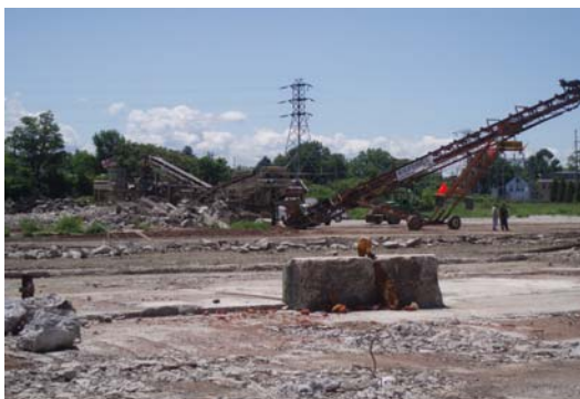
During remediation: Concrete crushing during Phase II remedial activities
