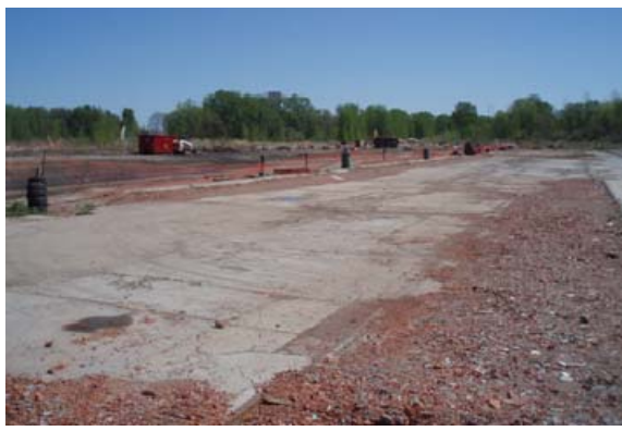
During remediation: Southwest corner after building demolition
