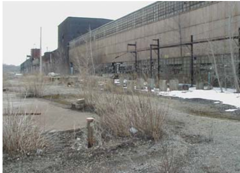
Before remediation: Northwest side of building
