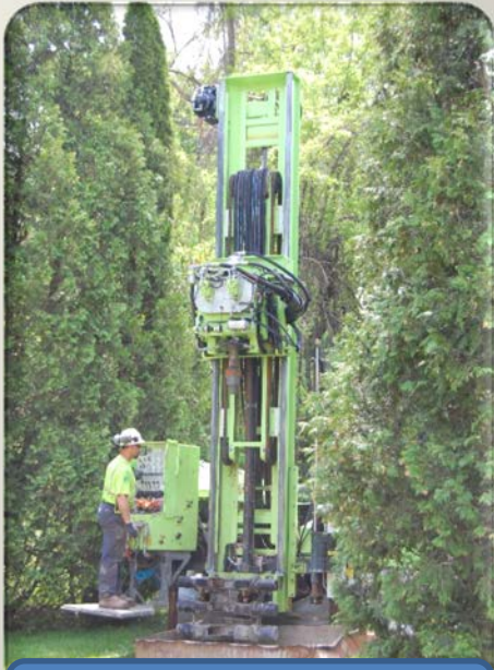
Photo 1: Rotary Vibratory Drill Rig Well Installation at John Street
