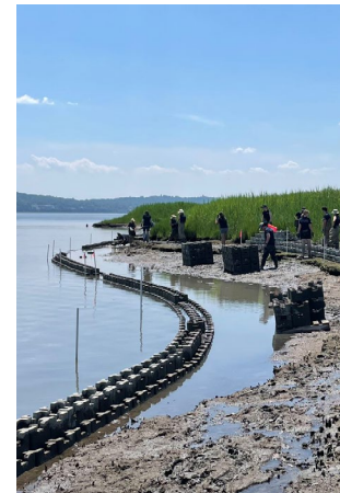
More than 8,000 oyster castles, each weighing 35 pounds, have been installed entirely by hand at low tide to construct the two intertidal sills. These castles installed here are not intended to support oyster settlement and growth, but sediment accretion.
