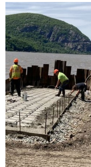
Installing shoreline stabilizers at Dockside Park in the Hudson Highlands.
