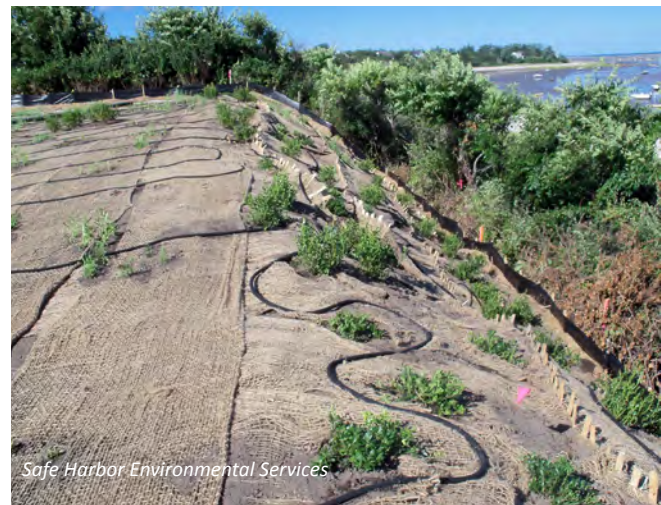
Erosion control blankets stabilizing a slope
