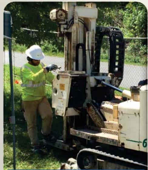
Photo 2: Direct push rig – soil and groundwater sampling at John Street
