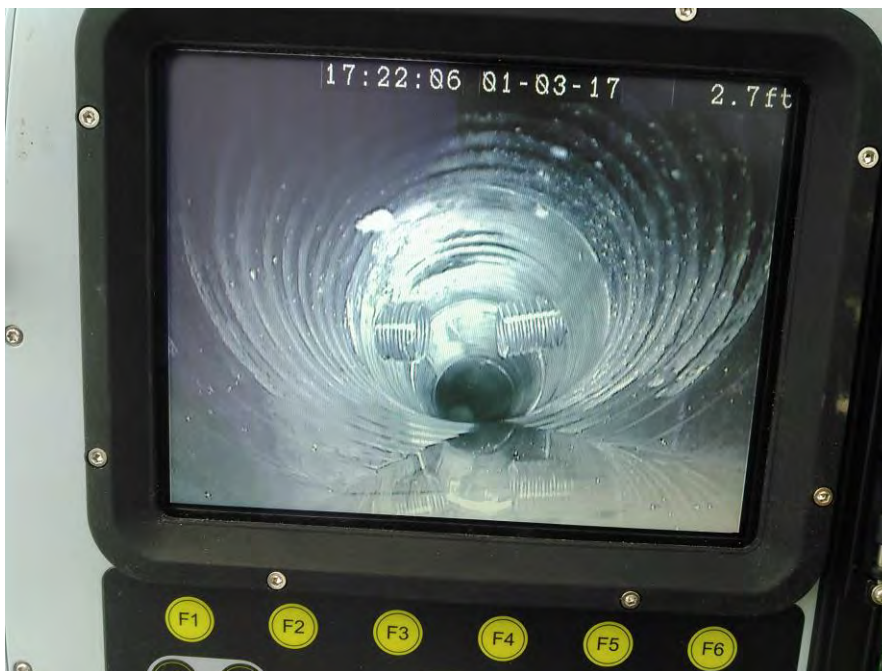
Picture of the 18 inch HDPE drain pipe from the courtyard into the building. Foundation drain pipes are shown entering the pipe.
