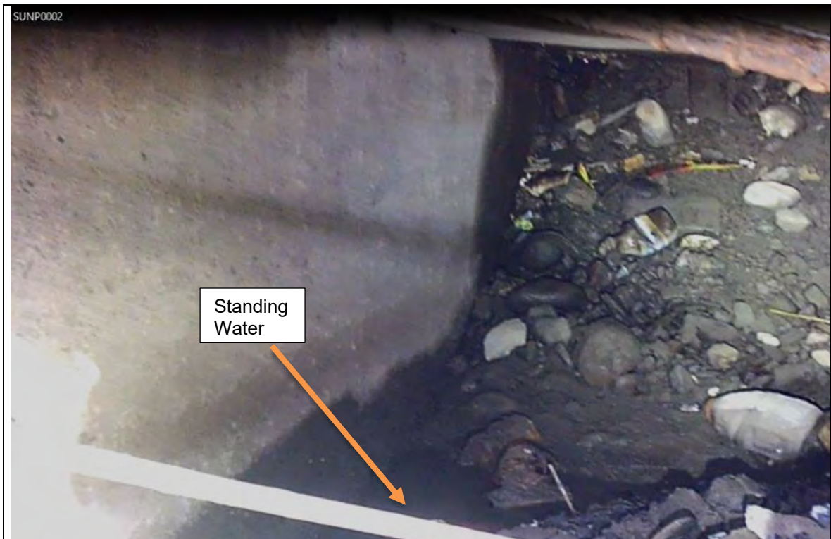
Photograph: 5 | Box Culvert Interior – Photo taken from open excavation looking north (towards Sand Bar) into northwest lower corner of structure.
