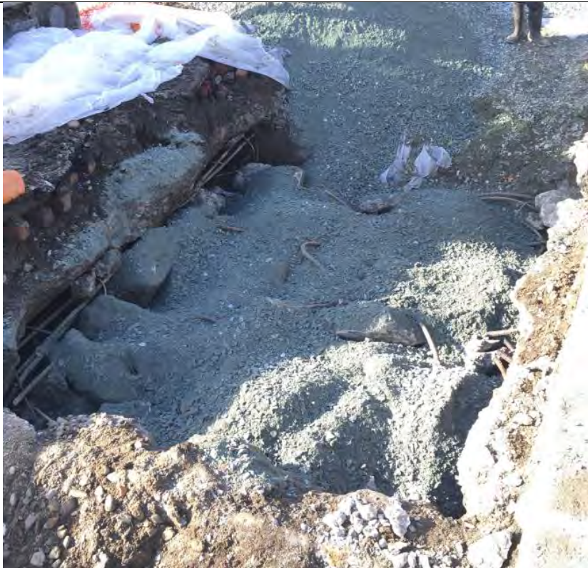
Photograph: 8 | Box Culvert – View facing west after addition of crusher run filling rubble voids
