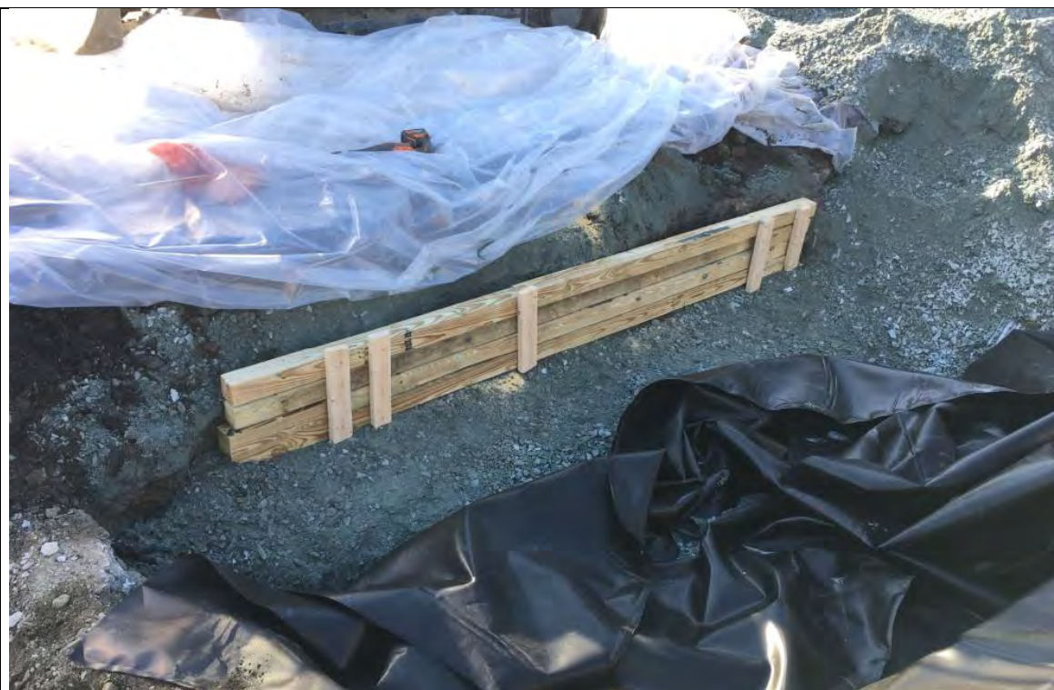
Photograph: 9 | Box Culvert – View facing southwest depicting timber supports
