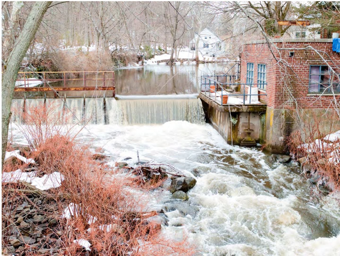
Flooding on the Sparkill Creek.
