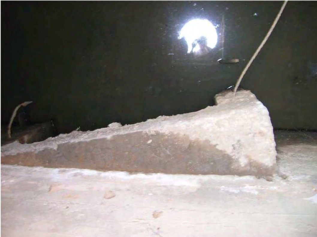
Picture #5- Looking down inside Oil Skimmer at ~5'wide influent culvert from east
