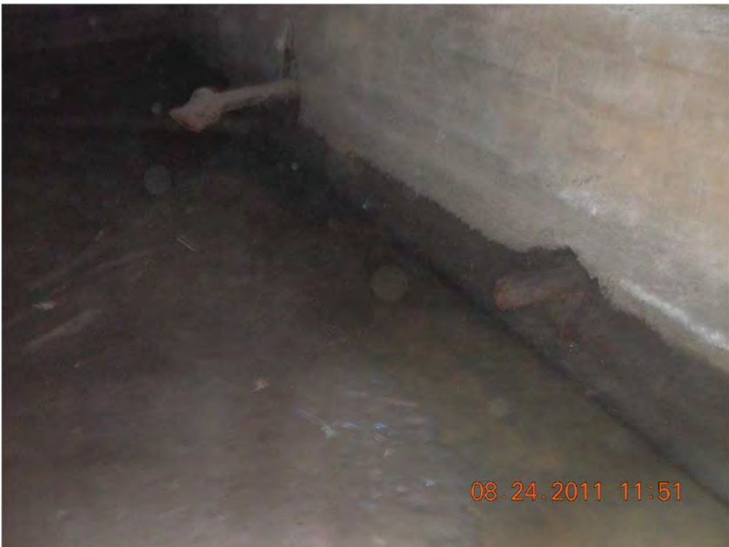
Picture #4- Inside Oil Skimmer from manhole looking NW at pipe penetrations
