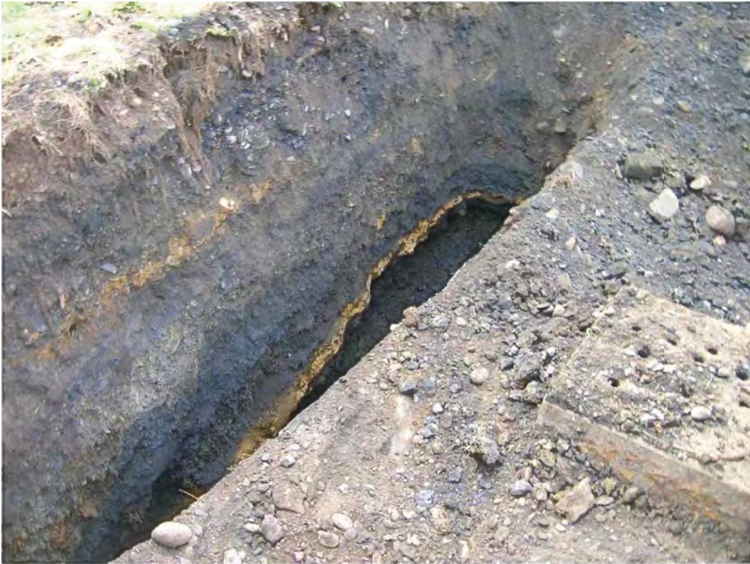
Picture #3- Test Pit #3, next to Oil Skimmer manhole
