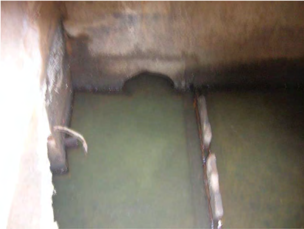
Picture #7- Inside Oil Skimmer looking south at pipe opening to south
