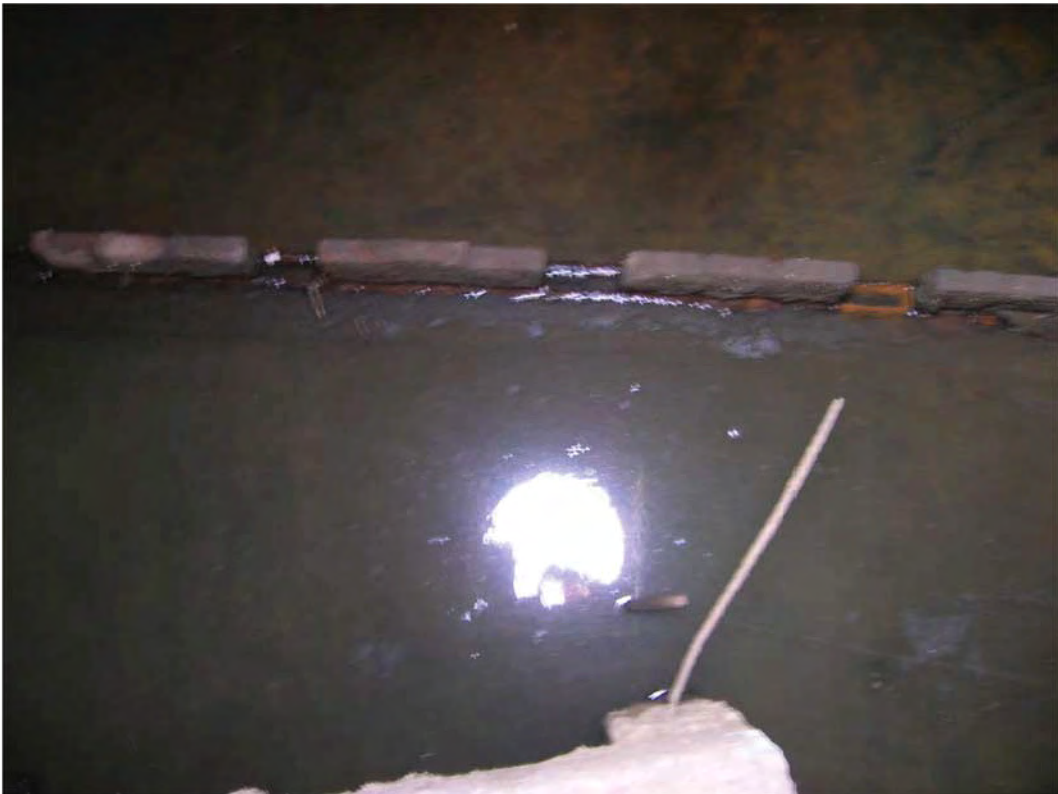
Picture #6- Looking down inside Oil Skimmer at internal baffles
