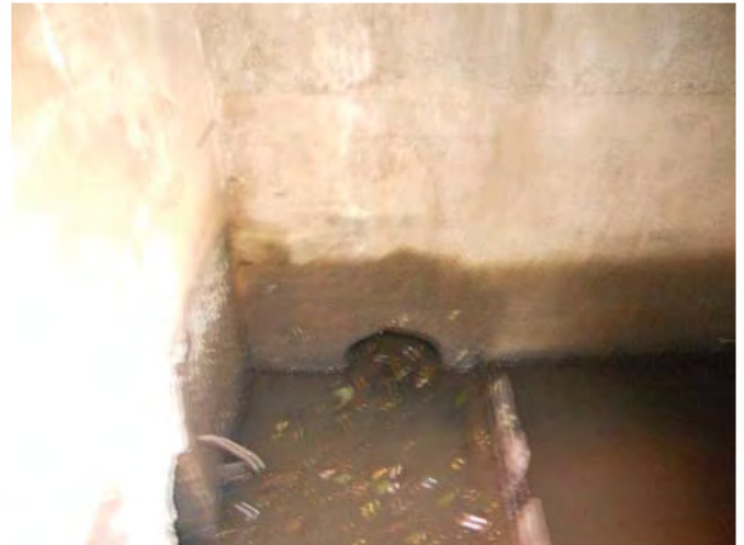
Inside OS2 view of 3x3 concrete encased pipe
