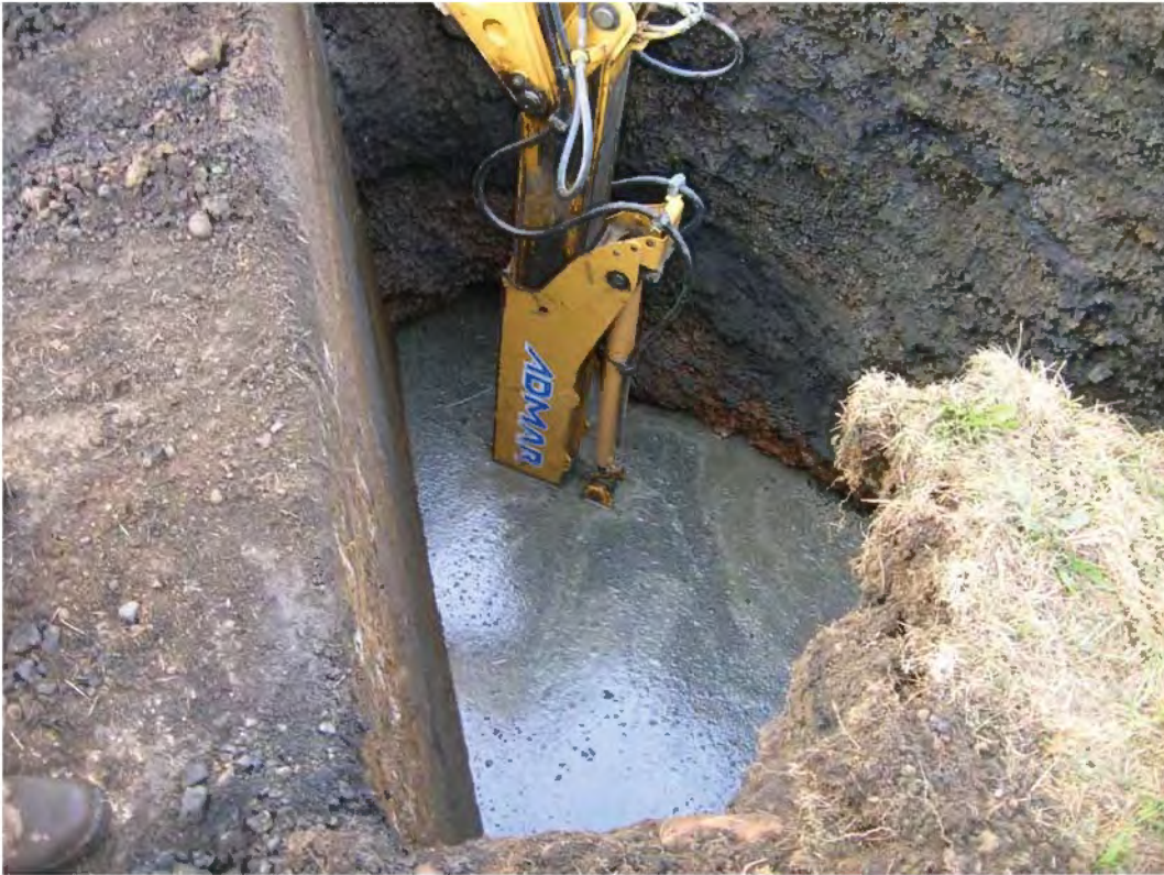
Picture #1- Test Pit #2
