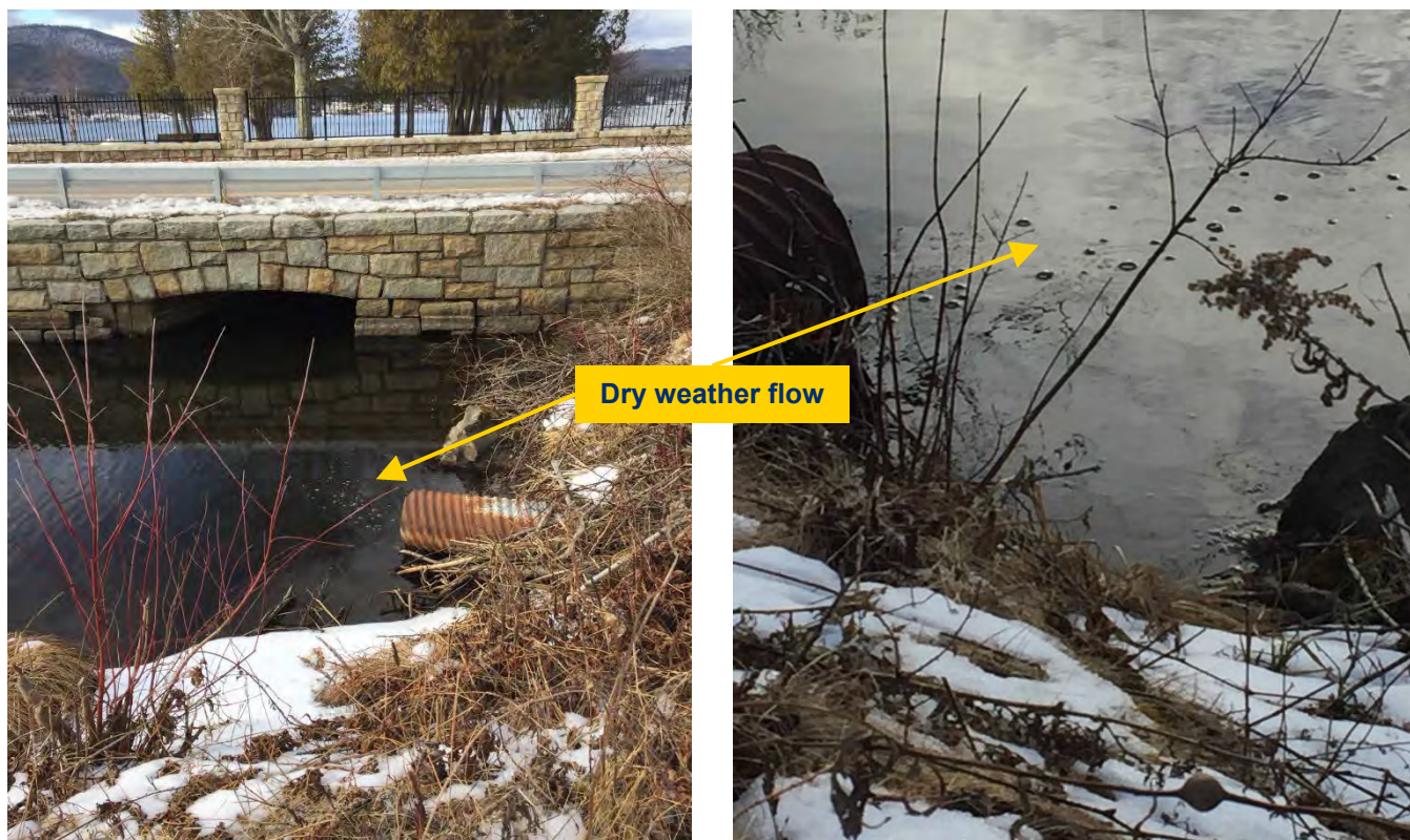
Figure B10. Photos of dry weather flows from 24" corrugated metal pipe into East Brook (photos taken January 28, 2017)
