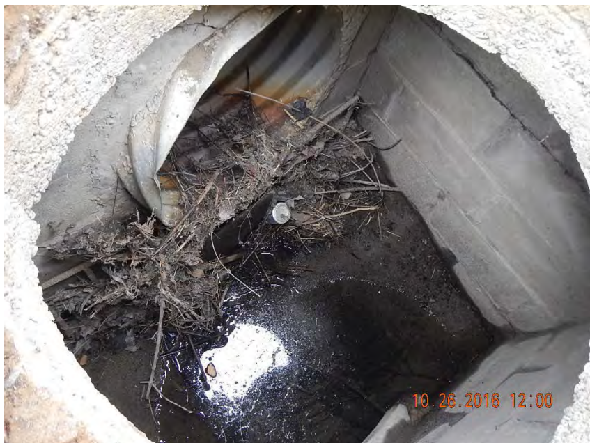
Figure B9. Photo of Cedar Lane Manhole with 24" corrugated metal pipe
