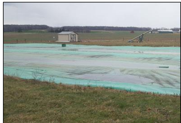
Manure storage with a cover and flare system
