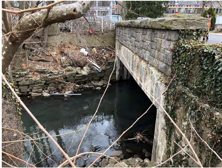
Figure 4-34: Looking at the Orchard Avenue upstream bridge face
