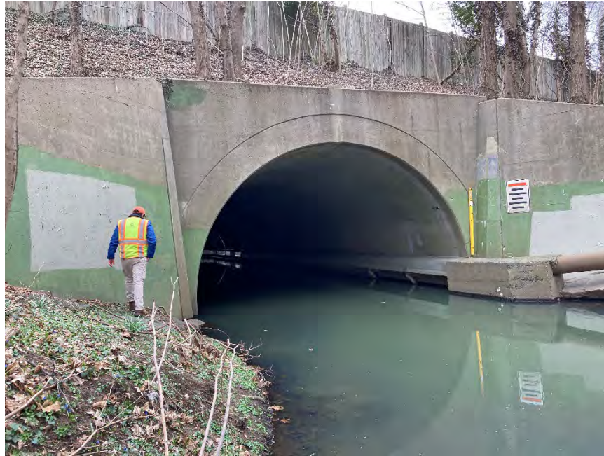
Figure 4-47: Looking downstream at the Metro-North/I-95 bridge
