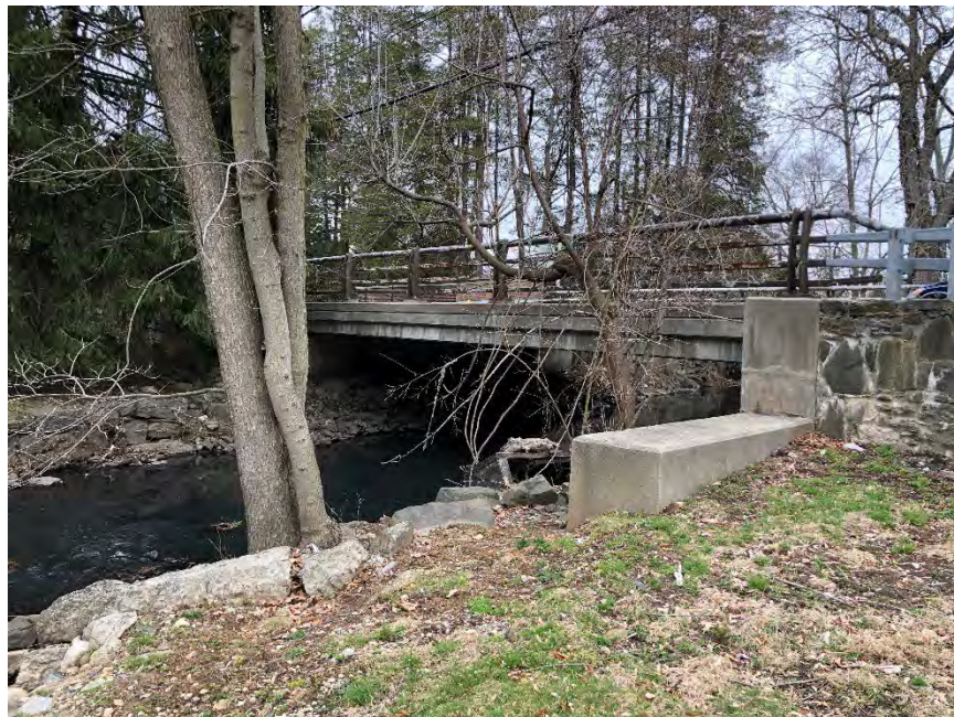
Figure 4-61: Looking upstream at the Purchase Street bridge
