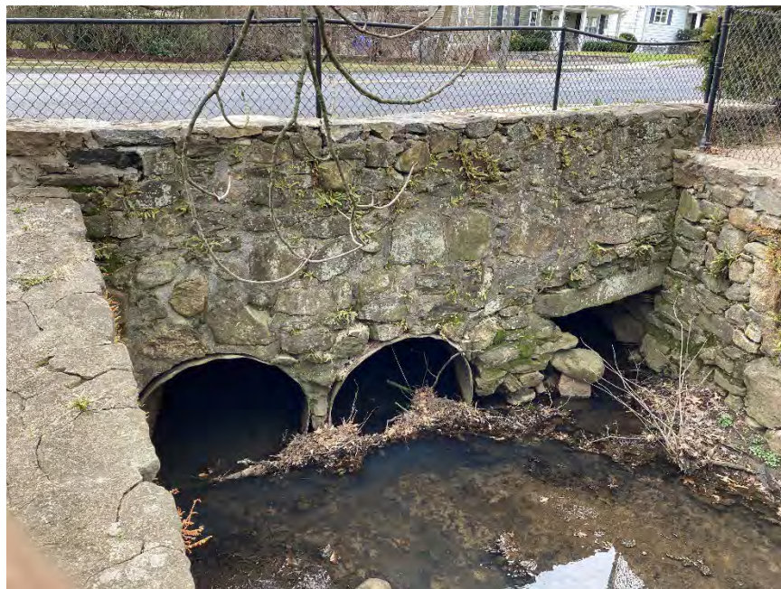
Figure 4-79: Looking downstream at the culvert structure under Betsy Brown Road
