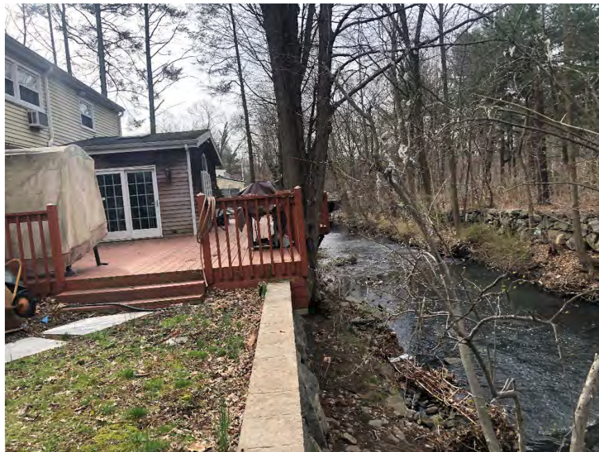
Figure 4-64: Blind Brook as it flows adjacent to homes on Brook Lane
