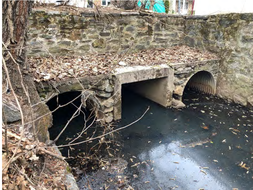
Figure 4-78: Looking upstream at the culvert structure under Argyle Road
