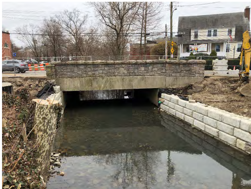
Figure 4-36: Looking downstream at the Locust Avenue bridge
