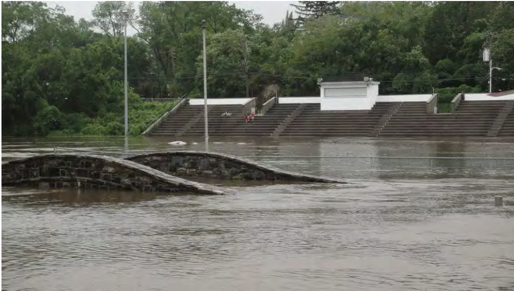
Figure 4-11 Rye High/Middle School football field flooded during Hurricane Irene 2011. The masonry stone arch bridge over Blind Brook is seen underwater (center left). Photo Courtesy of Patch.com News Report.
