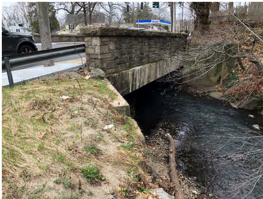
Figure 4-37: Looking downstream at the Theodore Fremd Avenue bridge
