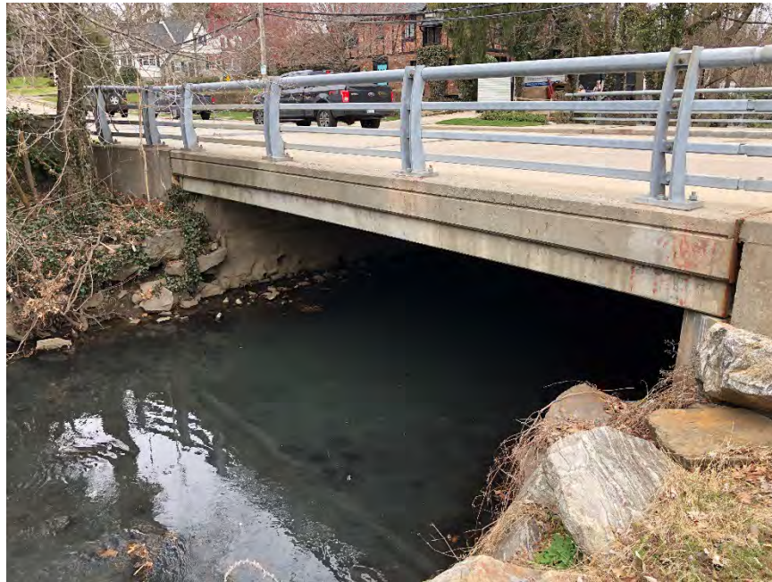
Figure 4-54: Looking upstream at the Highland Avenue bridge
