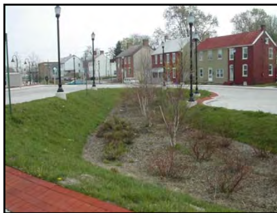
Figure 36: Example of a Bioretention Facility Along Roadway
