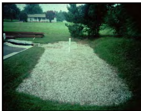
Figure 39: Infiltration Trench (Source: MA EOE, 2005)
