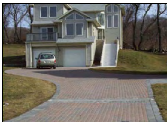
Figure 20: Permeable Pavers as an Alternative Driveway Surface (Source: MA EOEA, 2005)
