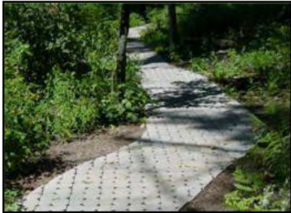
Figure 16: Sidewalk with a permeable paver surface (Source: MA EOEA, 2005)
