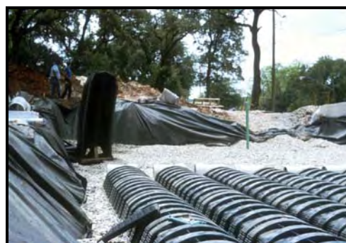
Figure 40: Infiltration Chambers (Source: MA EOE, 2005)
