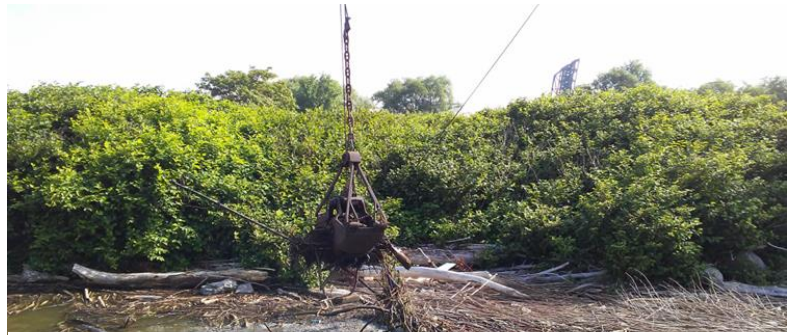
Figure 15. Three barges of large woody debris were removed from the “Blue Tower Turning Basin” site. The debris was removed from this site before in-water habitat was planted. A rootwad chain and floating boom system was then installed to deflect additional accumulation of debris.
