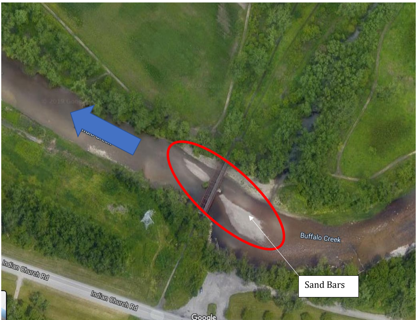
Figure 5. Sand Bar formation at the abandoned railroad bridge in the Town of West Seneca, NY.
