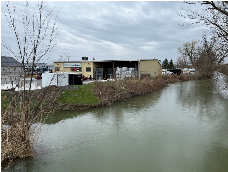
Photo D-4. Looking upstream toward Butternut Creek from the upstream face of the CSX railroad crossing. Photo taken 4/21/2022 by GSE.
