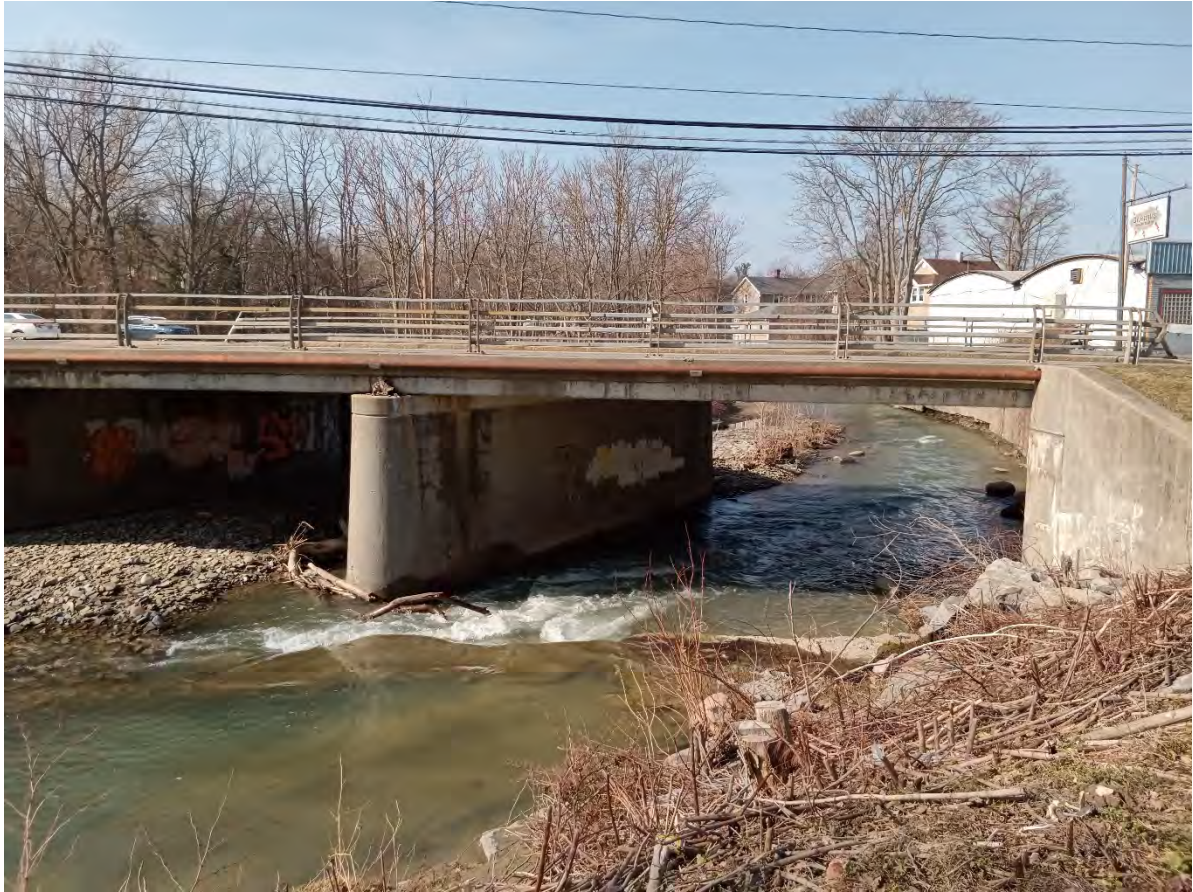
Figure 7-16. Water Street bridge, Fredonia, NY.
