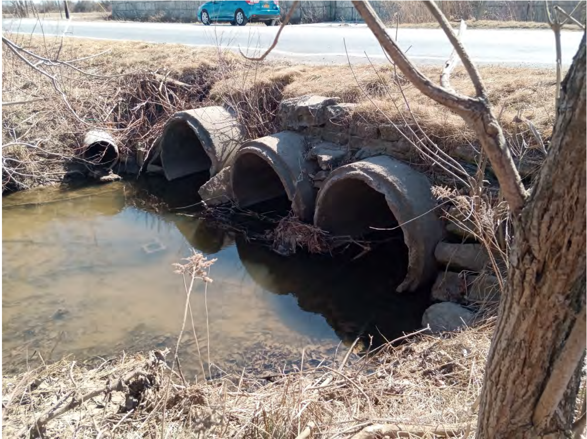
Figure 7-12. Cory Drive circular culverts, Wheatfield, NY.
