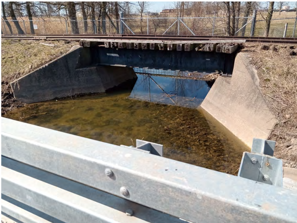
Figure 7-18. CSX Transportation railroad bridge crossing, Wheatfield, NY.
