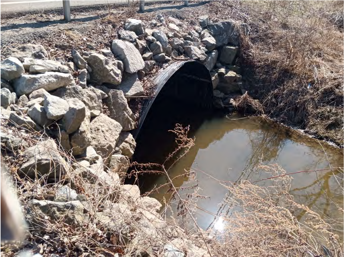
Figure 7-15. Downstream Walmore Road pipe culvert, Wheatfield, NY.
