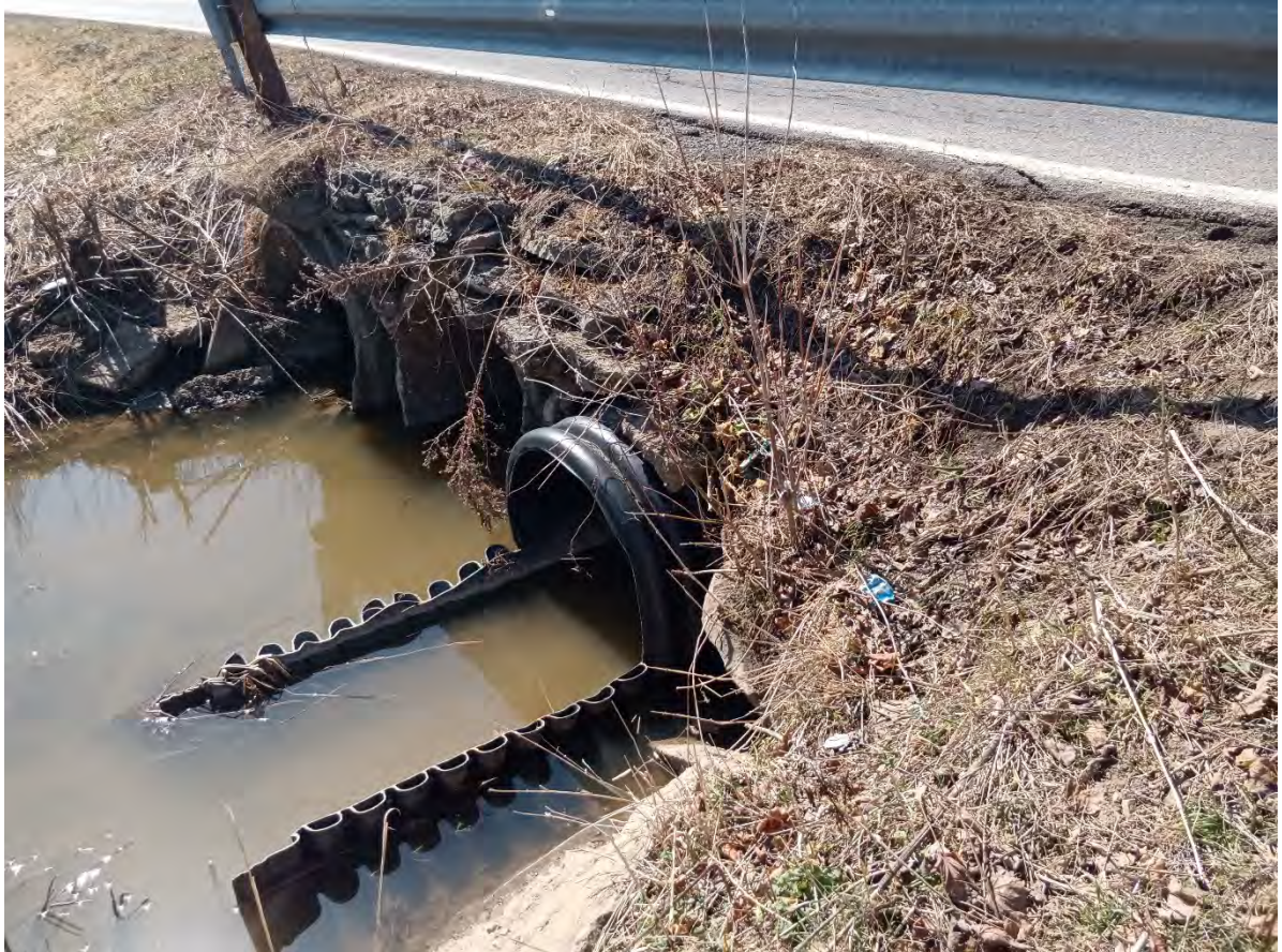
Figure 7-9. Upstream Walore Road circular culverts, Wheatfield, NY.
