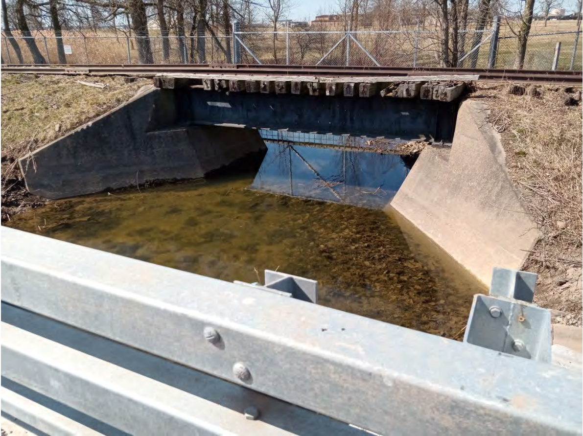
Figure 7-21. CSX Transportation railroad bridge crossing, Wheatfield, NY.
