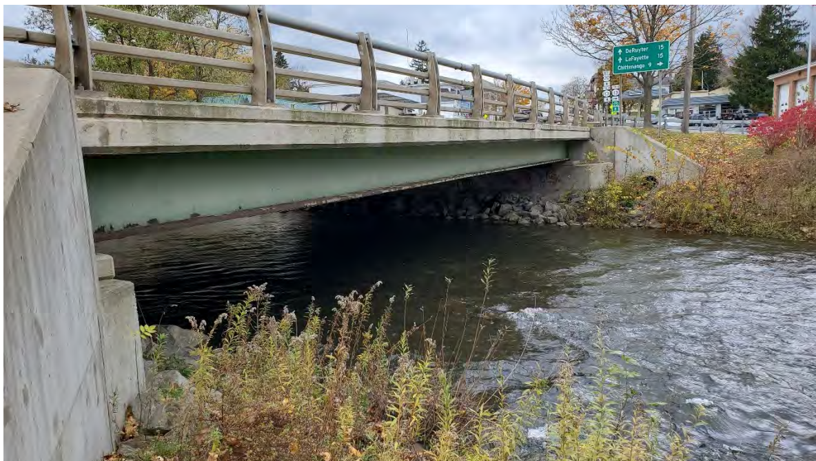
Figure 7-58. Albany Street/US-20 bridge, Cazenovia, NY.
