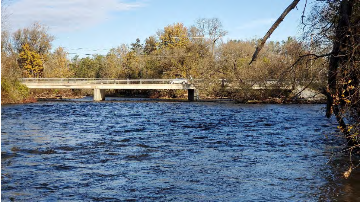
Figure 7-3. Lake Road/NY-31 bridge, Bridgeport, NY.
