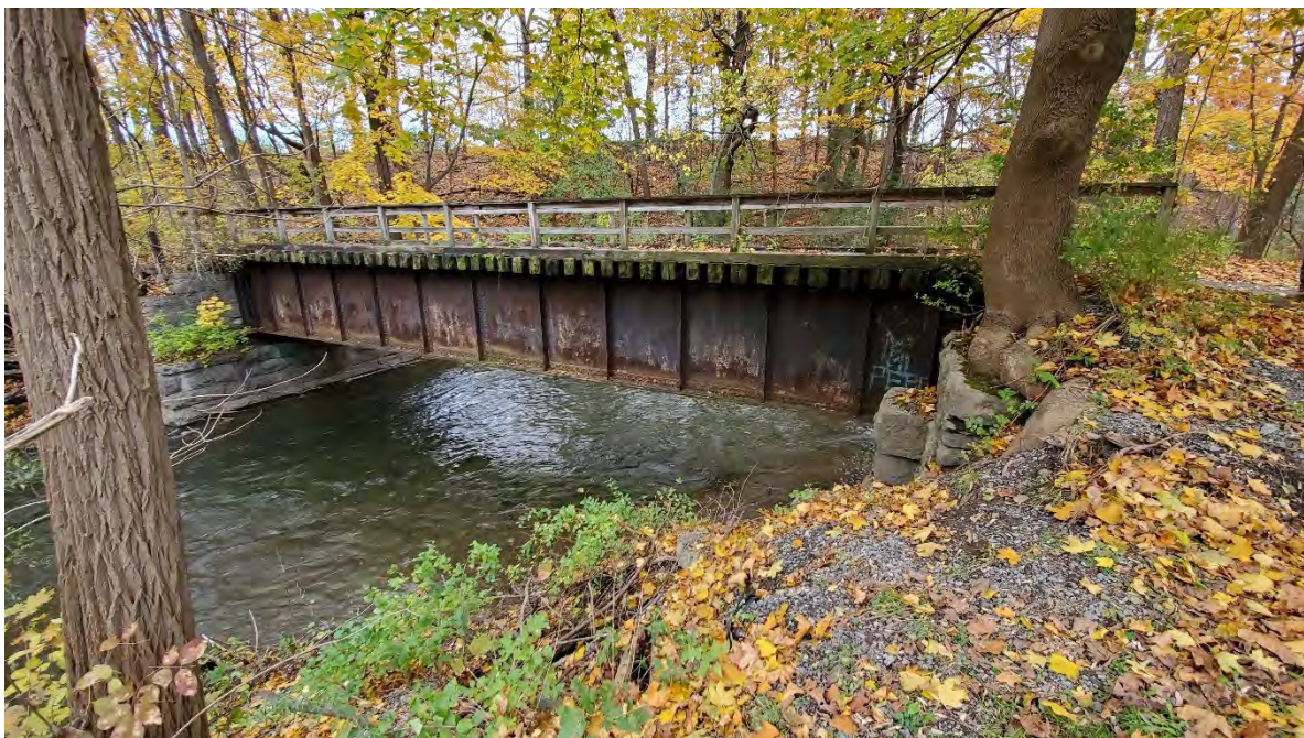
Figure 7-50. Chittenango Gorge Trail bridge, Cazenovia, NY.
