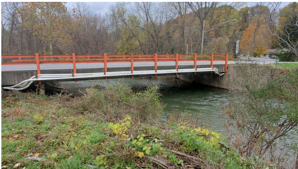
Figure 7-30. Tuscarora Road bridge, Chittenango, NY.
