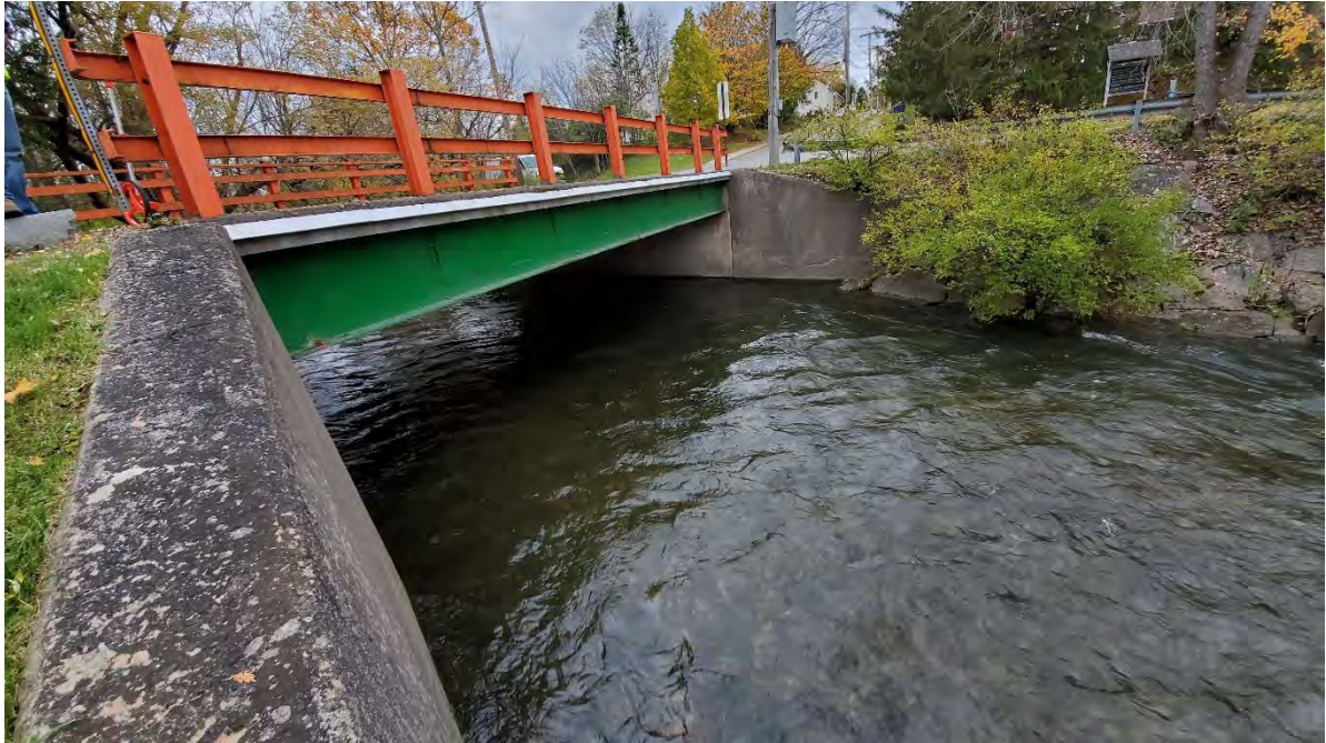
Figure 7-53. Burr Street bridge, Cazenovia, NY.
