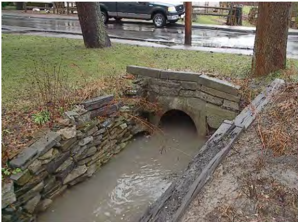
Figure 7-56. Burr Street culvert (Unnamed Tributary), Cazenovia, NY (MCEM 2016).
