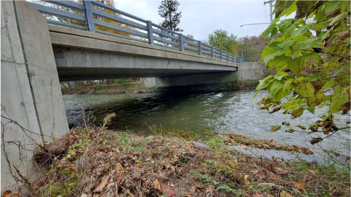
Figure 7-39. Madison Street bridge, Chittenango, NY.
