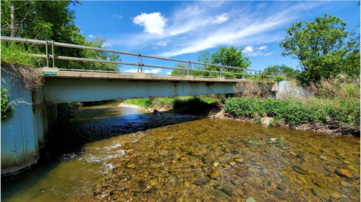
Figure 7-37. Jones Road bridge, Town of Freedom, NY.
