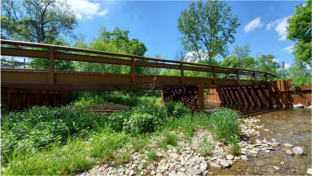
Figure 7-31. Sparks Road Bridge, Town of Freedom, NY.
