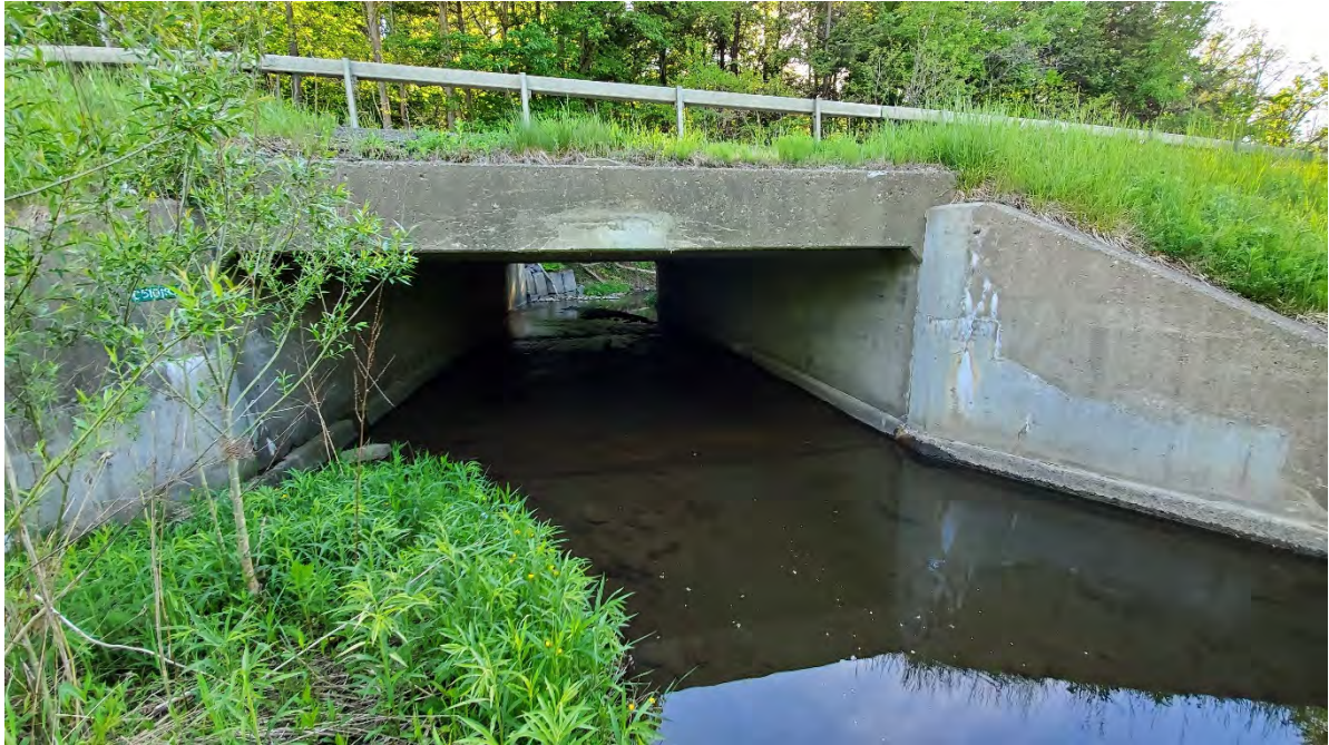
Figure 7-26. US-219 (3) culvert, Ashford, Cattaraugus County, NY.
