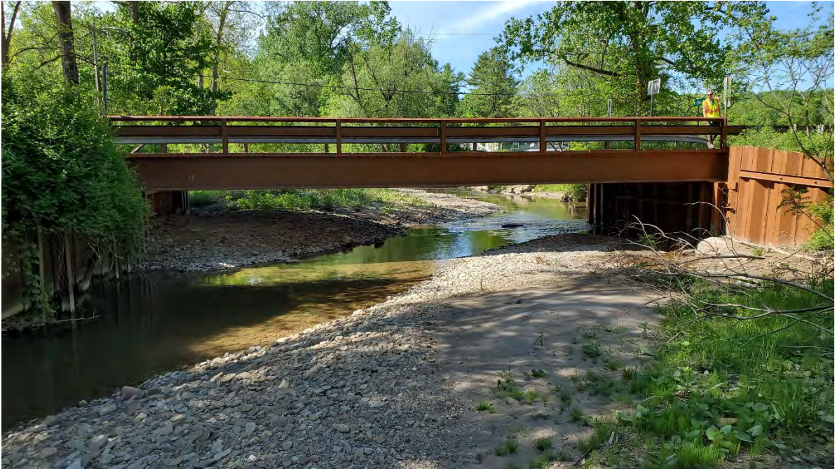
Figure 7-6. Hammond Hill Road bridge, East Otto, Cattaraugus County, NY.
