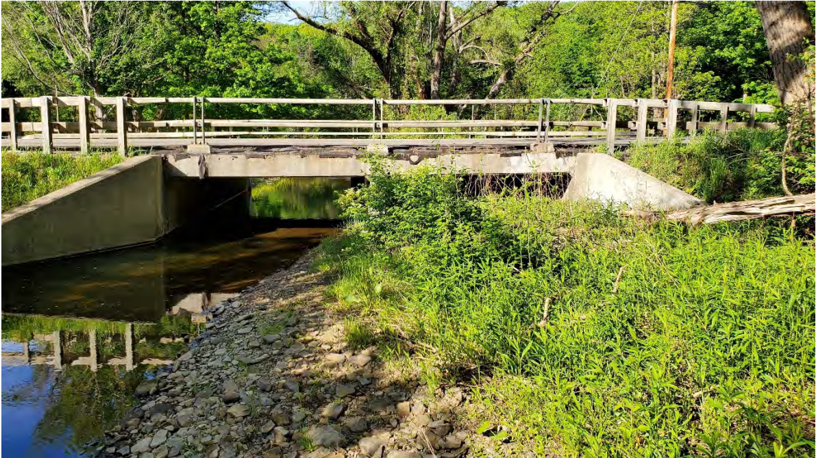
Figure 7-20. US-219 (2) bridge, Ashford, Cattaraugus County, NY.
