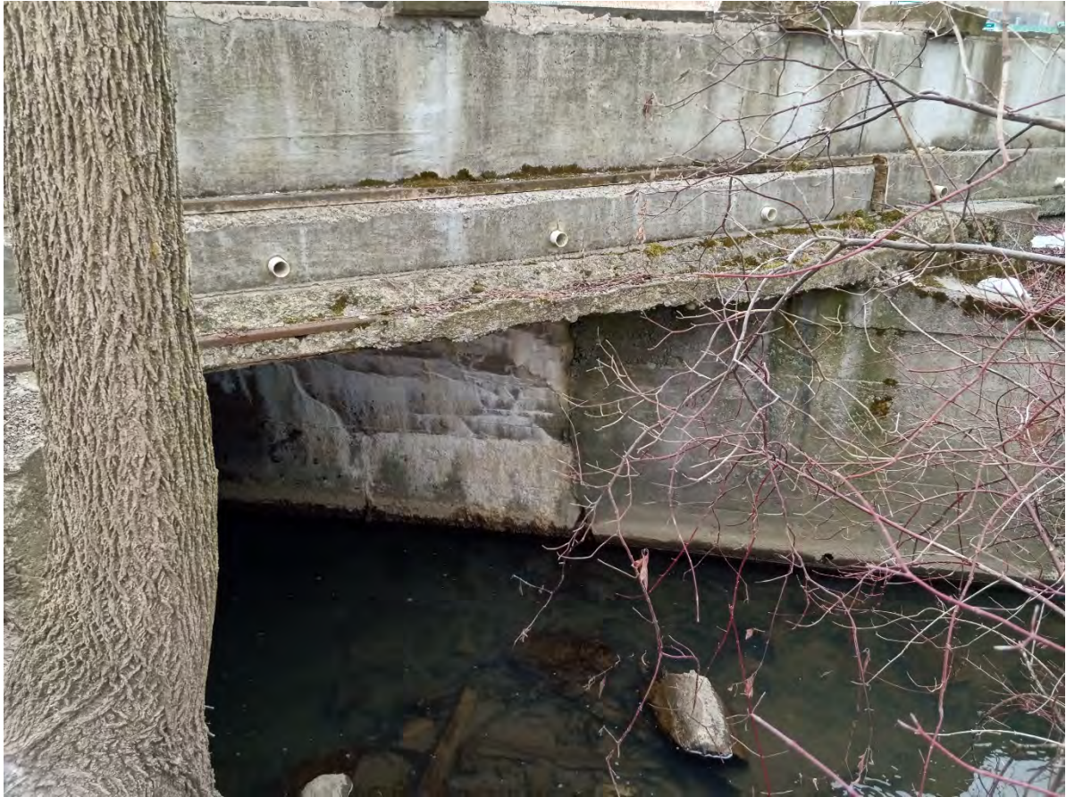
Figure 7-24. West Lucas Avenue culvert, Dunkirk, NY.
