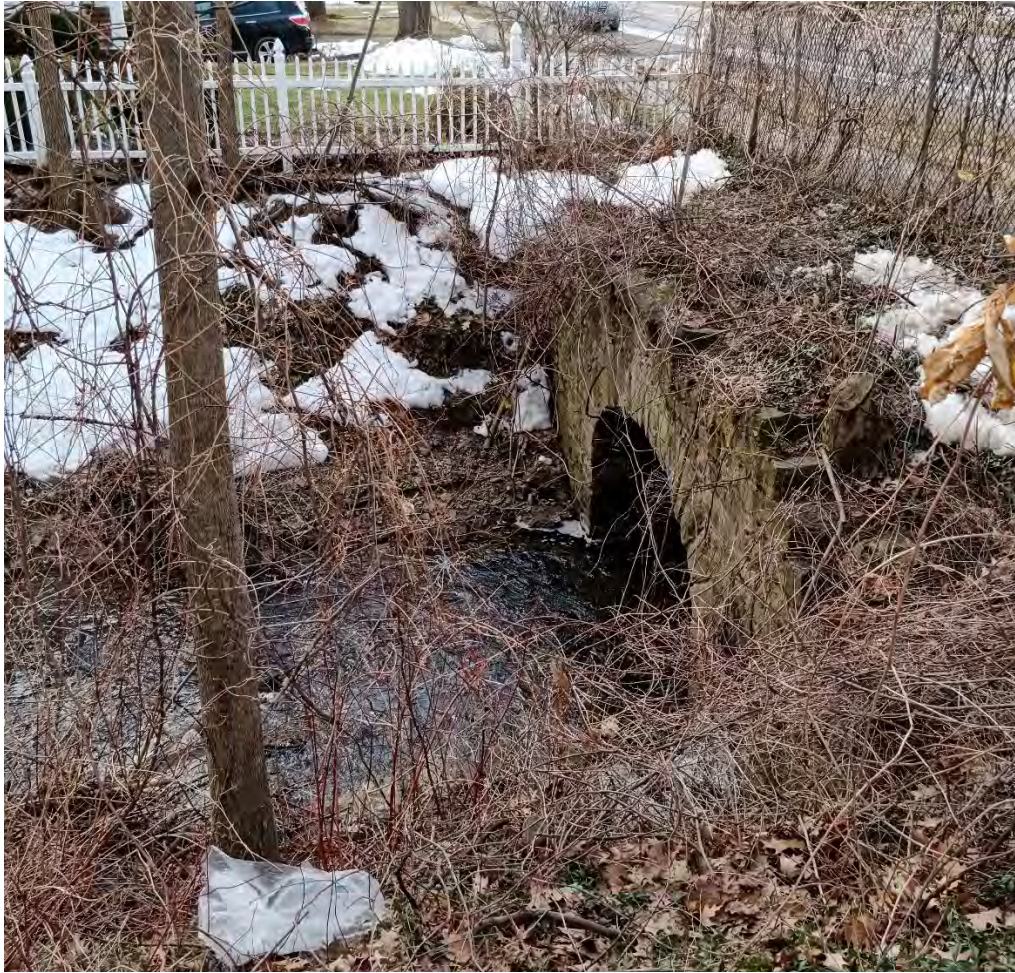
Figure 7-35. Central Avenue arch-culvert, Dunkirk, NY.
