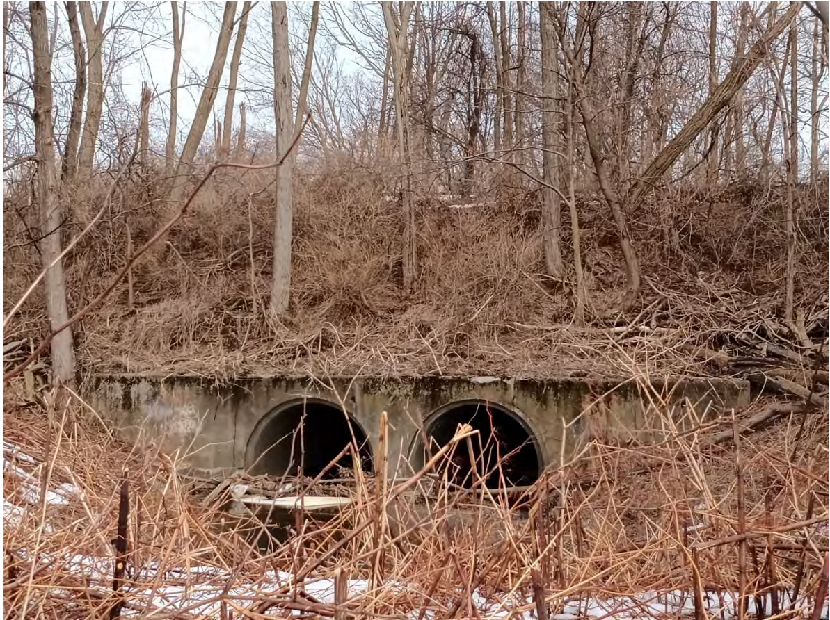
Figure 7-27. Norfolk And Western Railroad pipe culverts, Dunkirk, NY.
