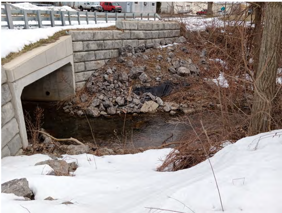
Figure 7-32. West Howard Avenue culvert, Dunkirk, NY.
