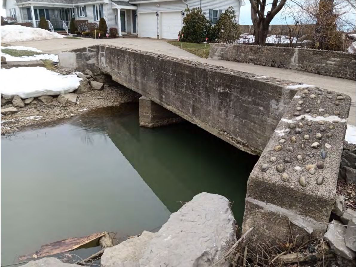
Figure 7-6. Crooked Brook Drive bridge, Dunkirk, NY.
