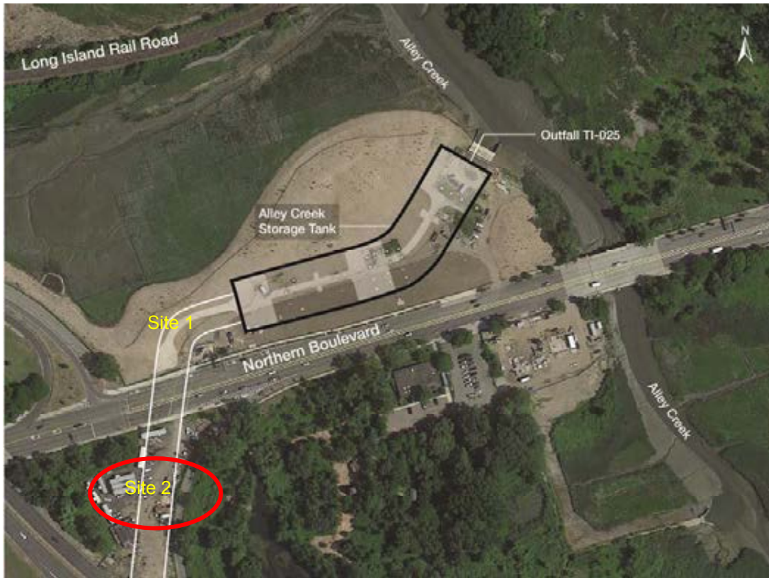
Figure 1. Alley Creek CSO Facility
