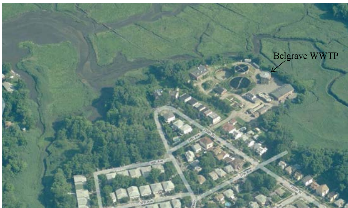
Figure 2-5. Location of the Belgrave WWTP, Adjacent to Udalls Cove (View NE)
