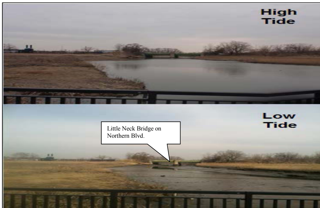
Figure 2. Looking North at Little Neck Bridge on Northern Boulevard
