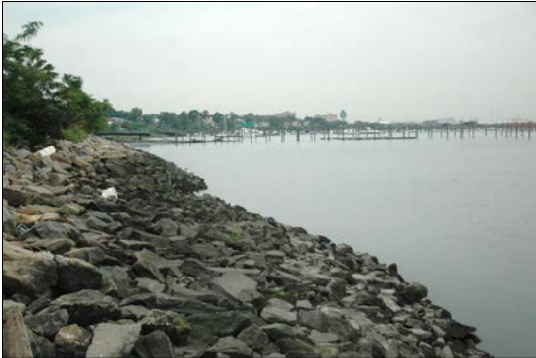
Figure 2-18. Rip-rap Shoreline View of Flushing Bay from Whitestone Expressway (Looking West)
