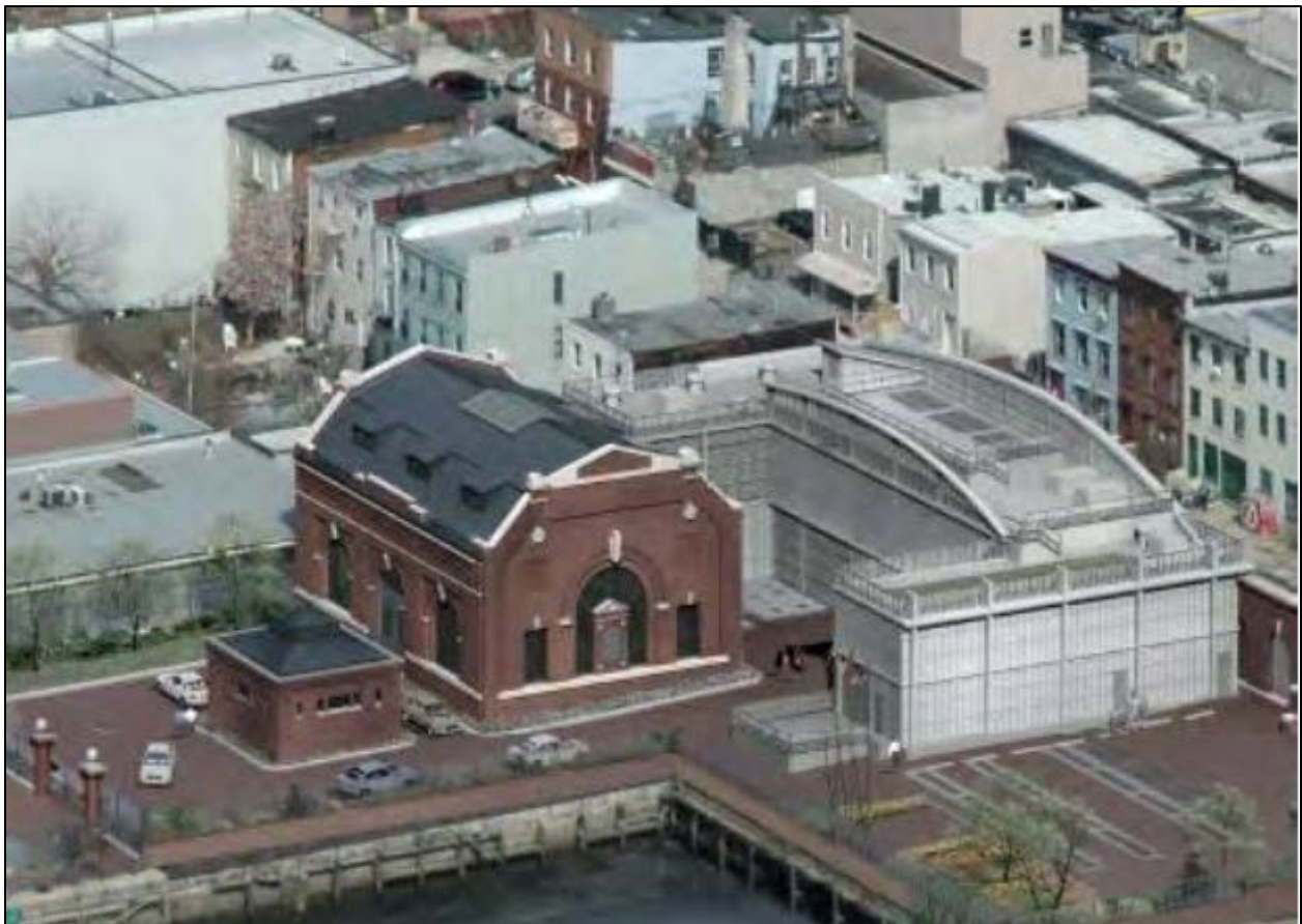
Figure 4-2. Rehabilitated Gowanus Pump Station at the Head End of Gowanus Canal
