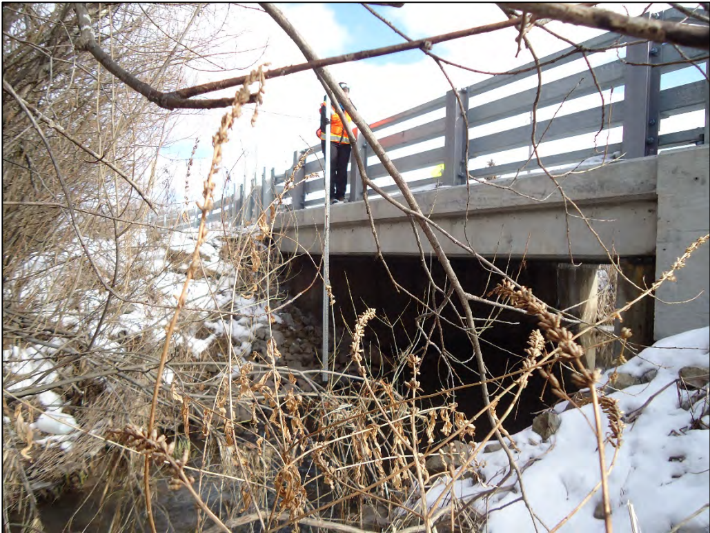
Photo C-6. Downstream Face of Locust Street bridge over Donner Creek (2/17/2020)
