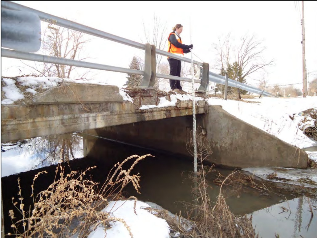
Photo C-3. Upstream Face of Hamm Road bridge over Donner Creek (2/17/2020)
