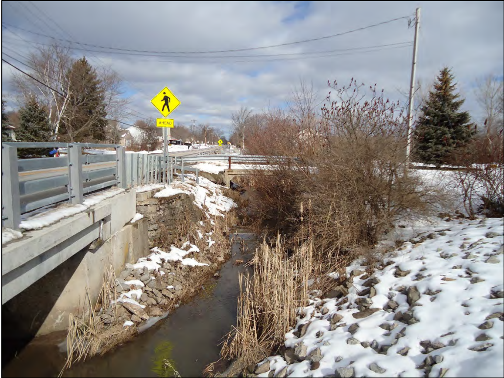
Photo C-5. Upstream Face of Locust Street bridge over Donner Creek (2/17/2020)
