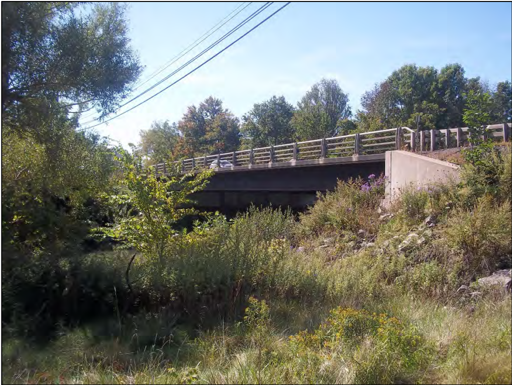
Photo C-7. Upstream face of Transit Road bridge crossing Tonawanda Creek (9/19/2019)
