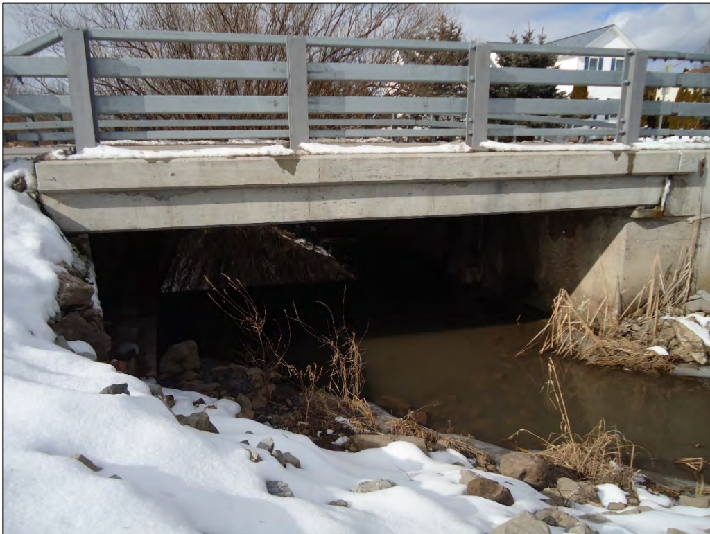
Photo 2: Upstream Face of Locust Street Bridge over Donner Creek
