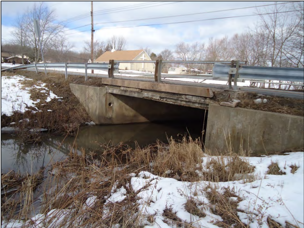
Photo C-4. Downstream Face of Hamm Road bridge over Donner Creek (2/17/2020)
