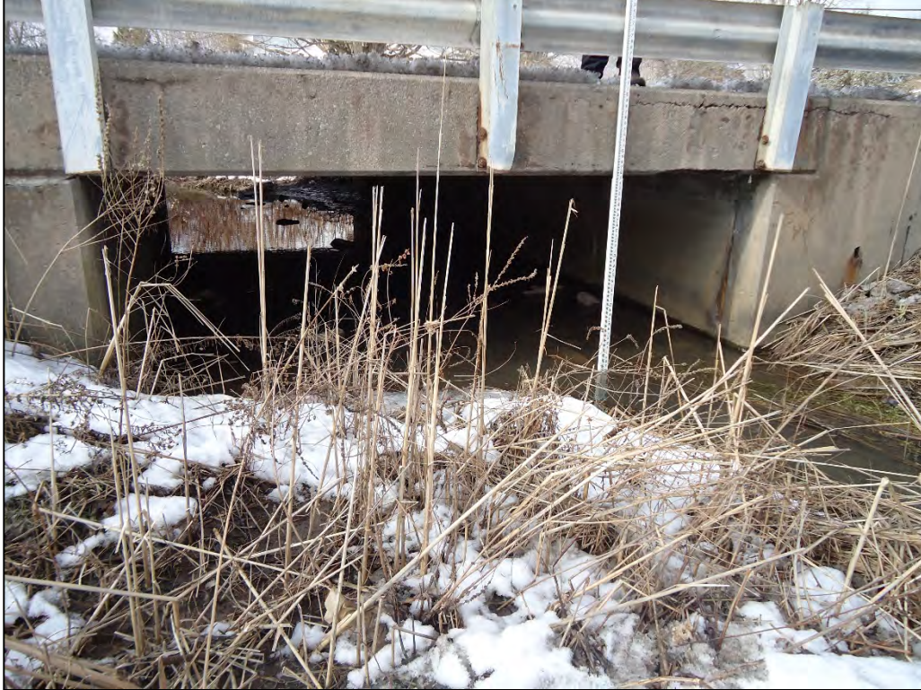
Photo C-1. Upstream face of Beattie Ave bridge crossing Donner Creek (2/17/2020)
