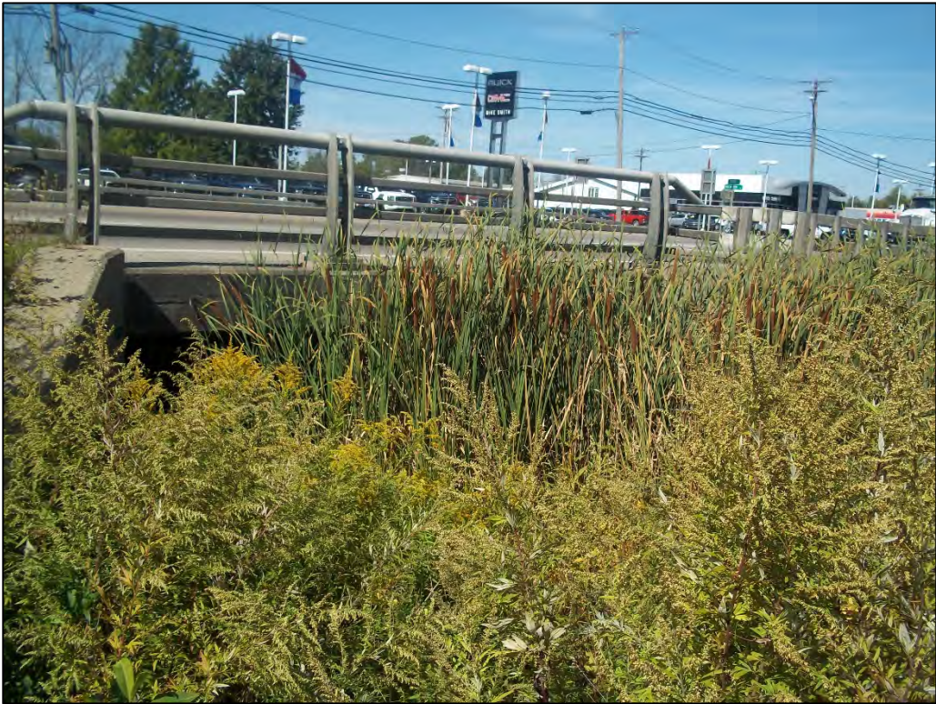
Photo C-8. Upstream face of Transit Road bridge crossing at Donner Brook (9/19/2019)
