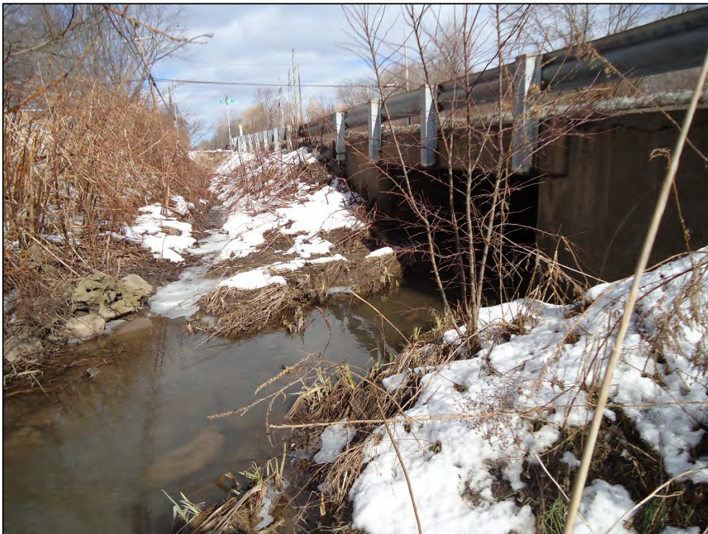
Photo C-2. Downstream face of Beattie Ave bridge crossing Donner Creek (2/17/2020)
