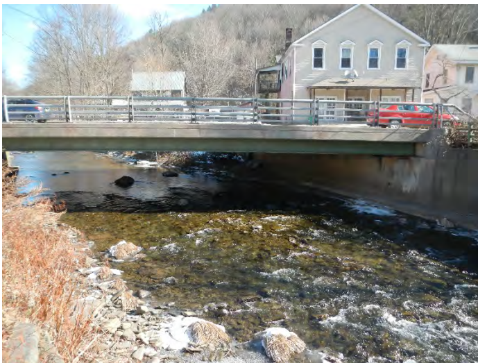
Photo 4-11 Routes 30/206 bridge over Downs Brook, Downsville
