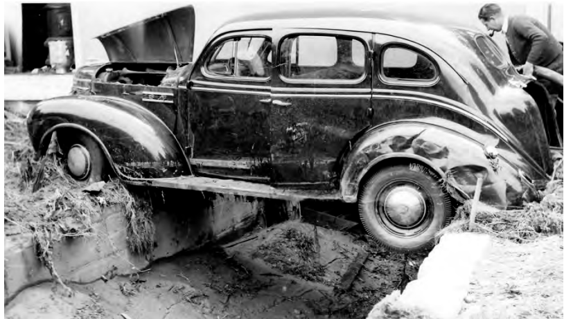
Photo 4-10 Flood damage in Downsville, 1942. Courtesy of Colchester Historical Society, Downsville, New York
