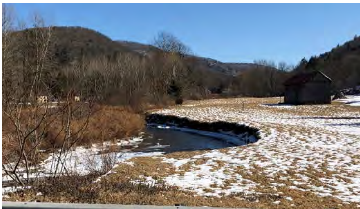
Photo 4-3 Bank Failure Upstream of Bodoit Road Crossing of Fish Creek
