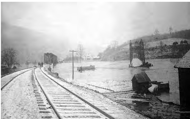
Photo 4-4 Fish's Eddy in 1903 flood. The railroad bridge is now the single-lane Route 28 bridge. The former road bridge is visible to the right; only substructural features remain today. Courtesy of Colchester Historical Society, Downsville, New York
