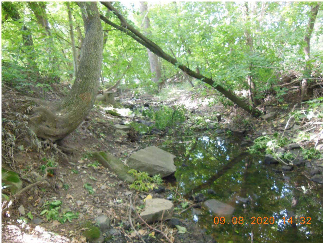
Photo D-6. Channel Viewed Upstream from Eighteenmile Creek Culvert Inlet
