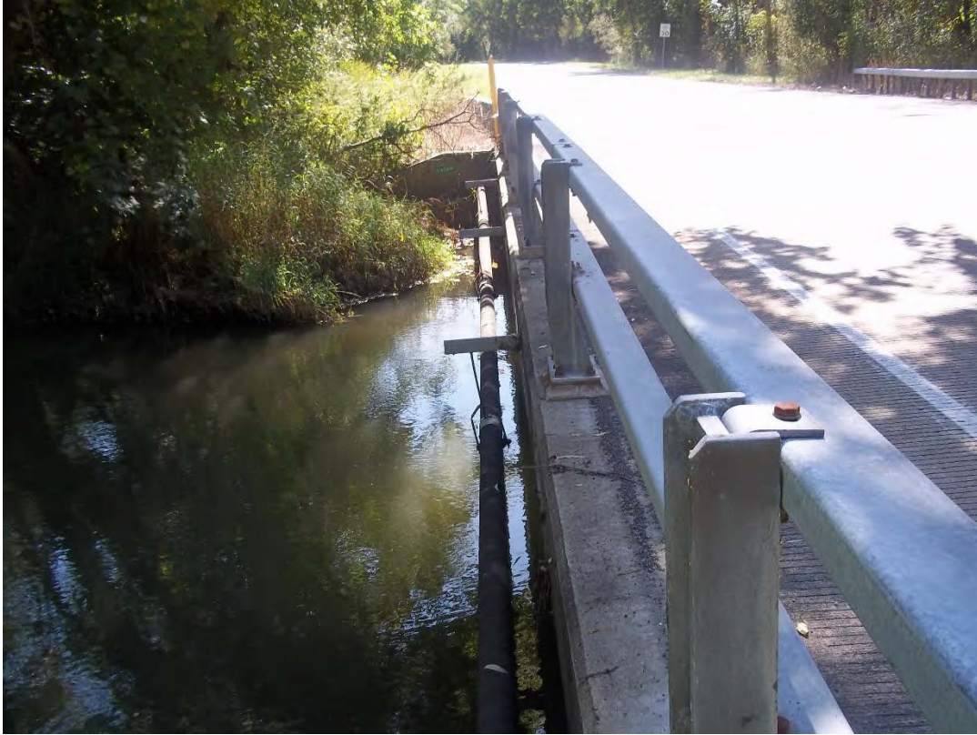
Photo D-3. Downstream Face of Plank Road Bridge
