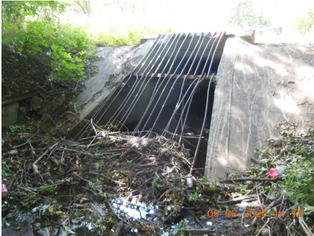
Photo D-5. Eighteenmile Creek Culvert Inlet
