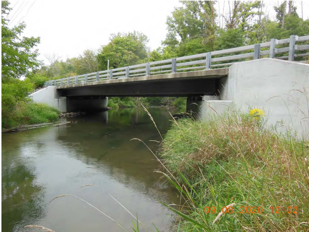
Photo D-1. Upstream Face of Stone Road Bridge
