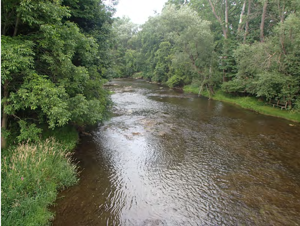
Photo D-3. Wehrle Drive looking upstream
