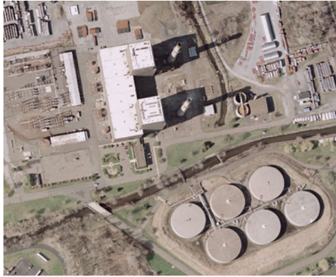
Mirant Bowline viewed from above
