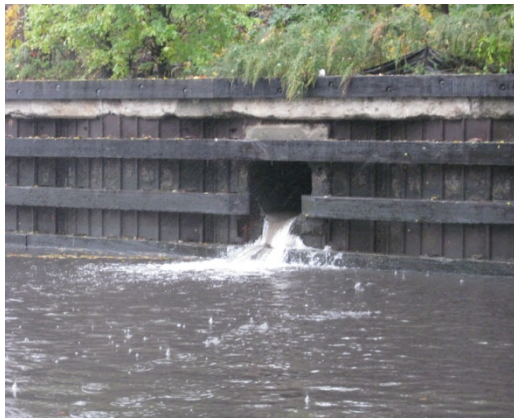
CSO on the Hutchinson River
