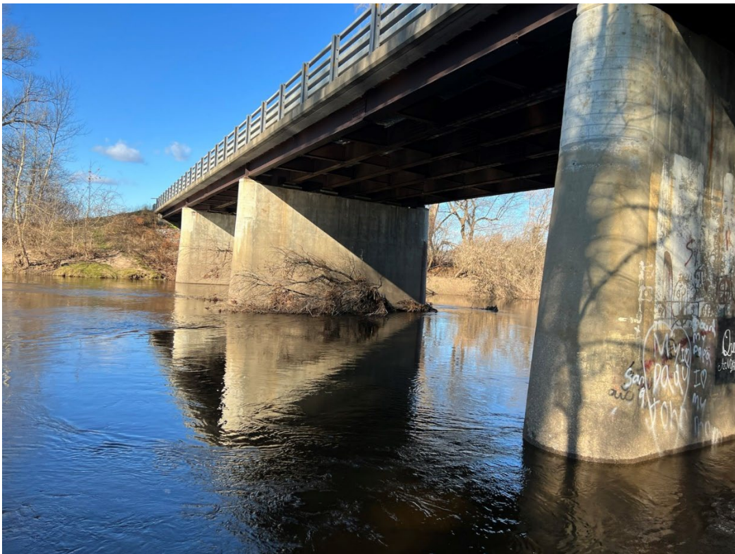
Photo D-4. Downstream Face of State Route 49 Bridge
