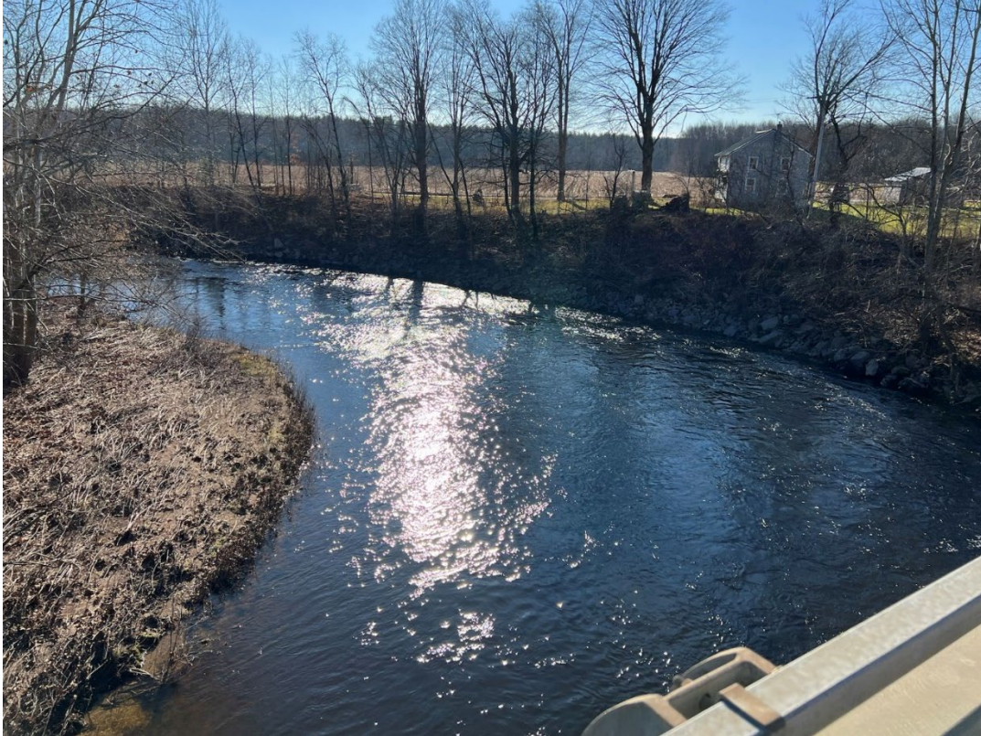
Photo D-7. Channel Downstream of Oswego Road Bridge
