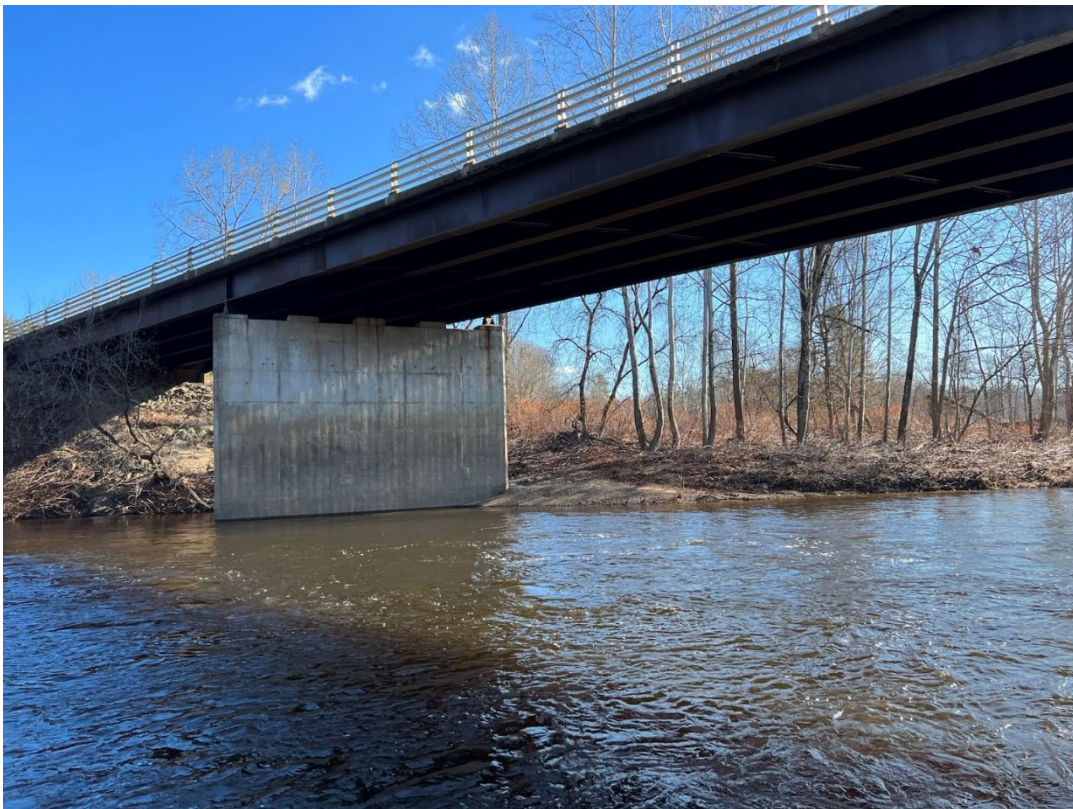
Photo D-6. Downstream Face of Oswego Road Bridge
