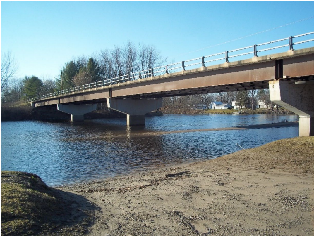
Photo D-1. Upstream Face of Higginsville Road Bridge
