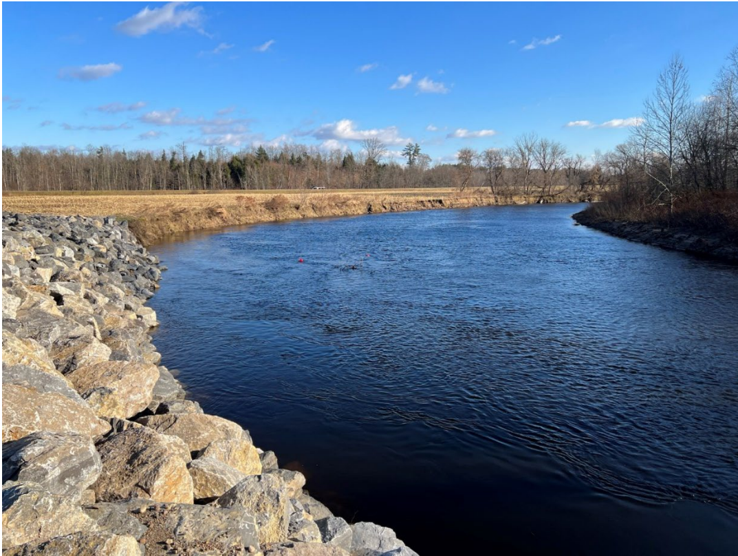
Photo D-3. Bank Stabilization near Old State Route 49 Looking Upstream
