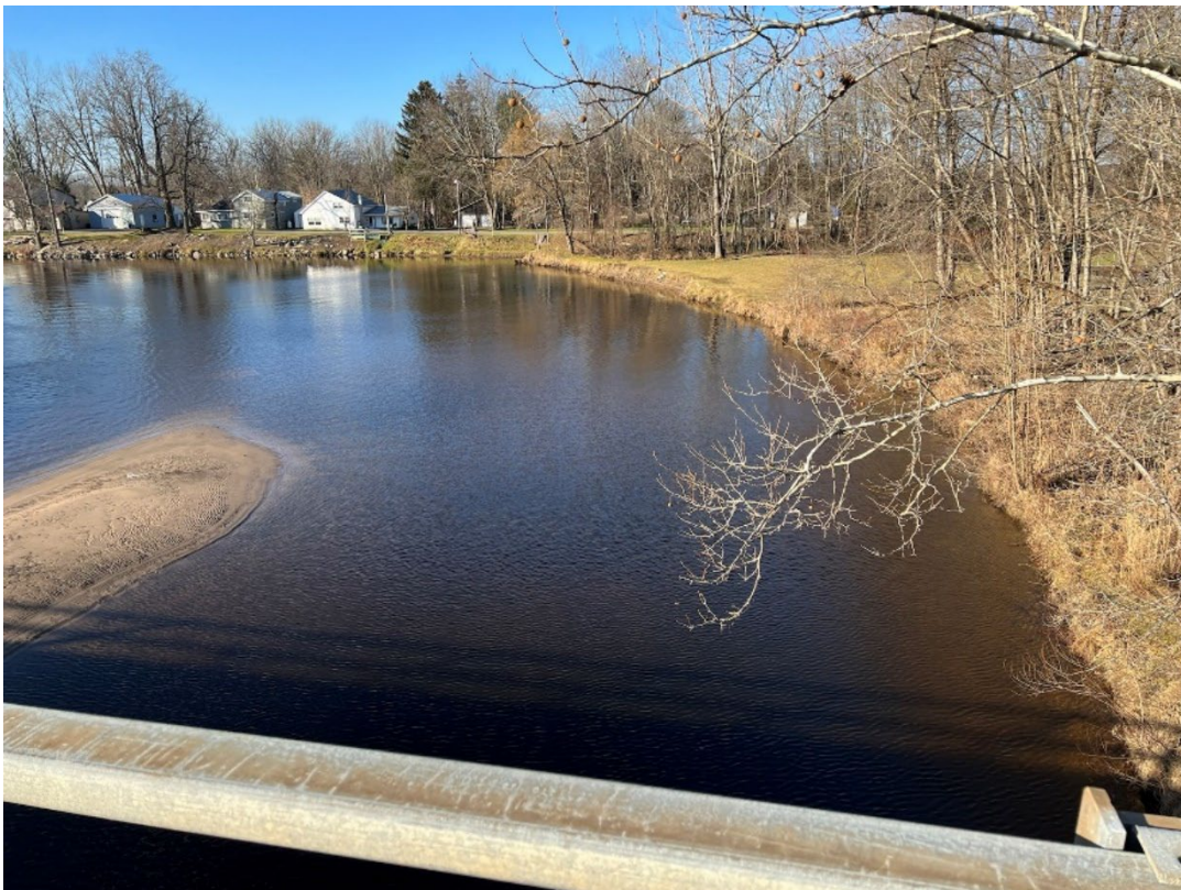
Photo D-2. Channel Downstream of Higginsville Road Bridge
