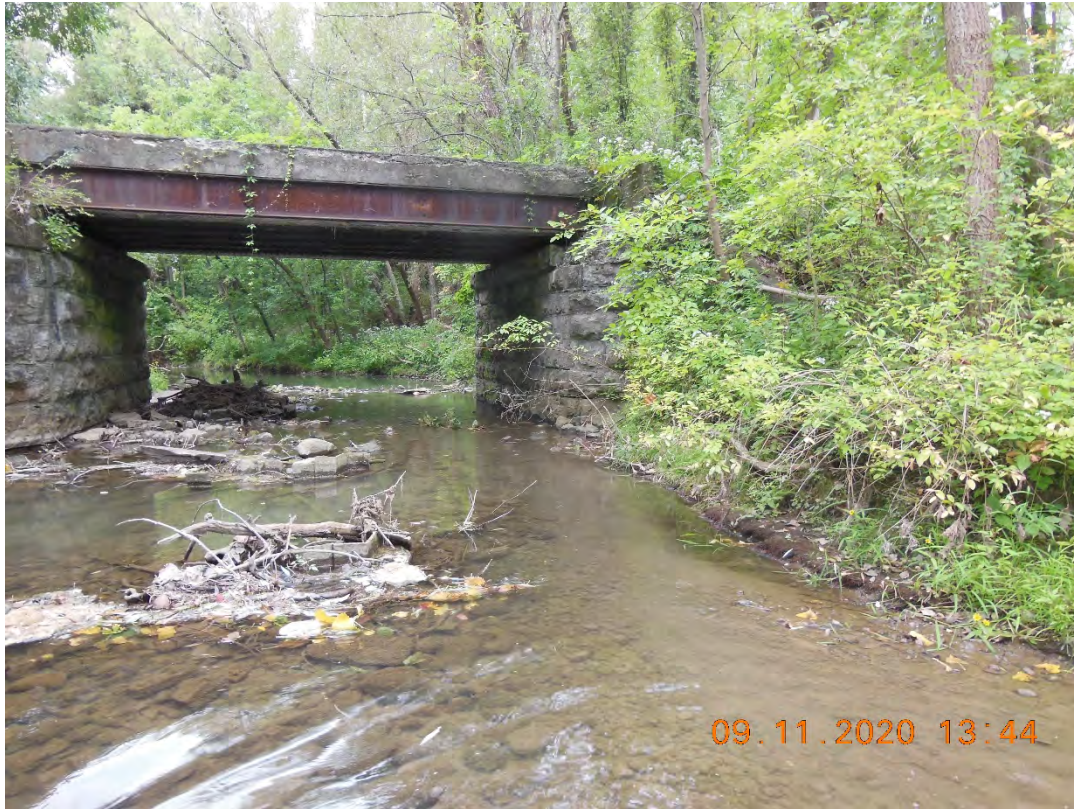
Photo D-7. Upstream Face of Peanut Line Bridge
