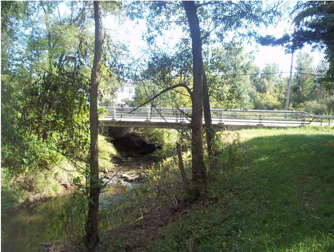
Photo D-3. Downstream Face of Casey Road Bridge
