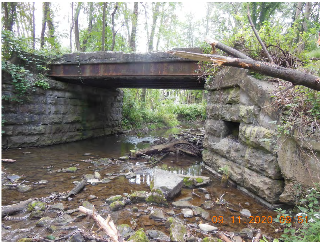
Photo D-8. Downstream Face of Peanut Line Bridge
