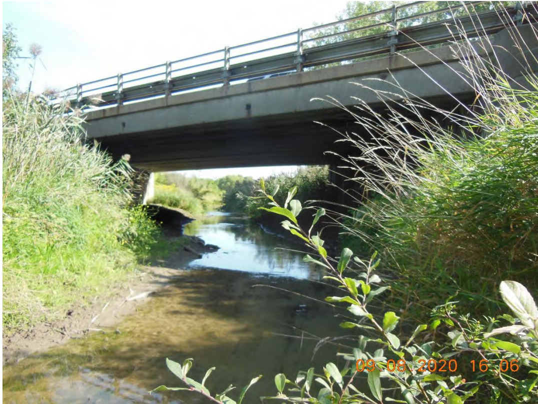
Photo D-1. Downstream Face of North French Road Bridge
