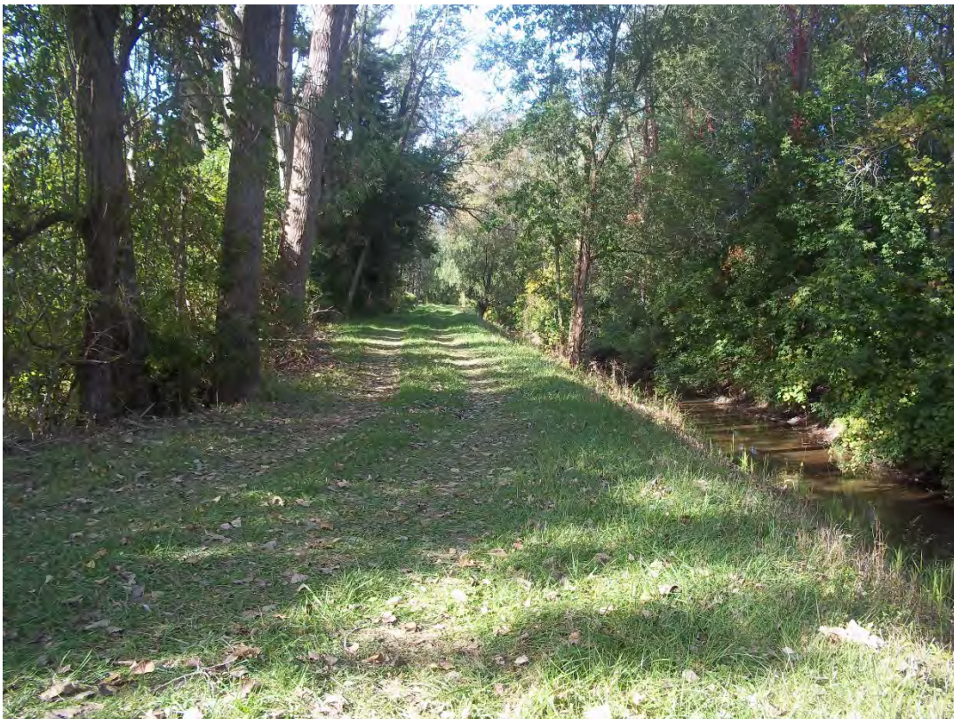
Photo D-6. Levee Downstream of Casey Road along Left Overbank
