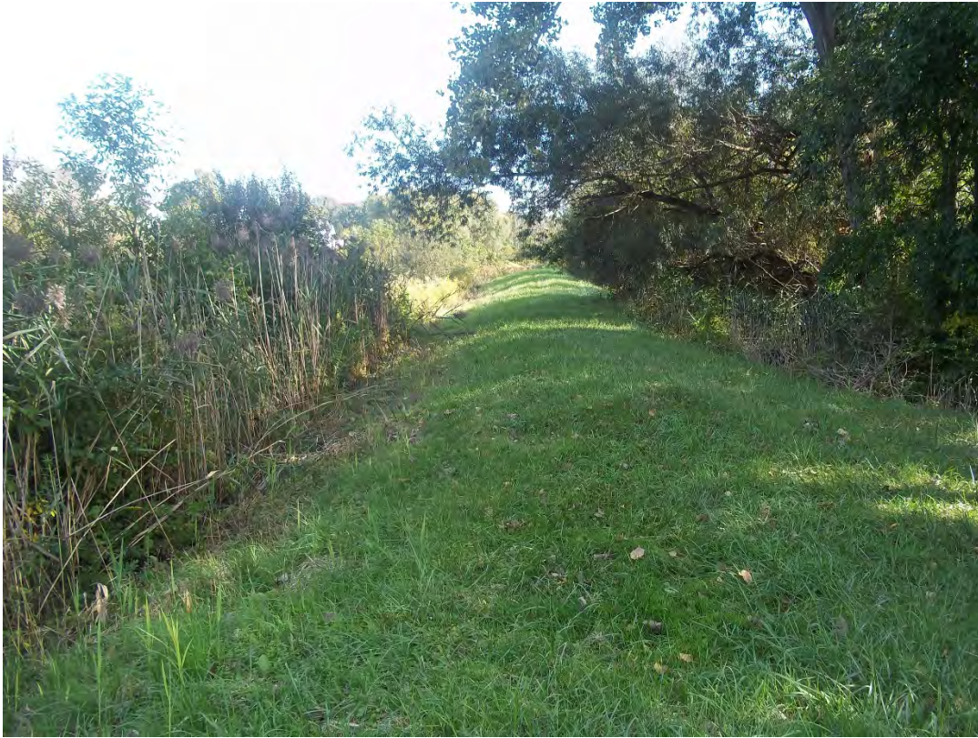
Photo D-5. Levee Upstream of North French Road along Left Overbank
