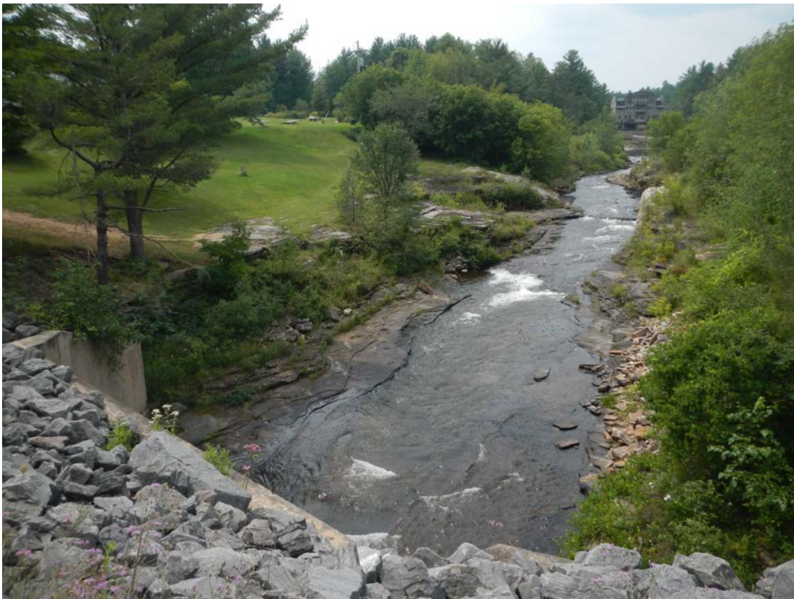
Figure 4-44: Devil's Den Road culvert crossing of the Great Chazy River. View is looking upstream from the culvert.
