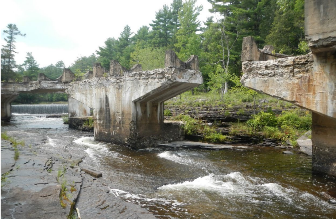
Figure 4-52: Concrete piers that formerly carried penstocks from McGregor Dam to McGregor Powerhouse were constructed in the river channel. Low-head dam is visible in background on left side of image.
