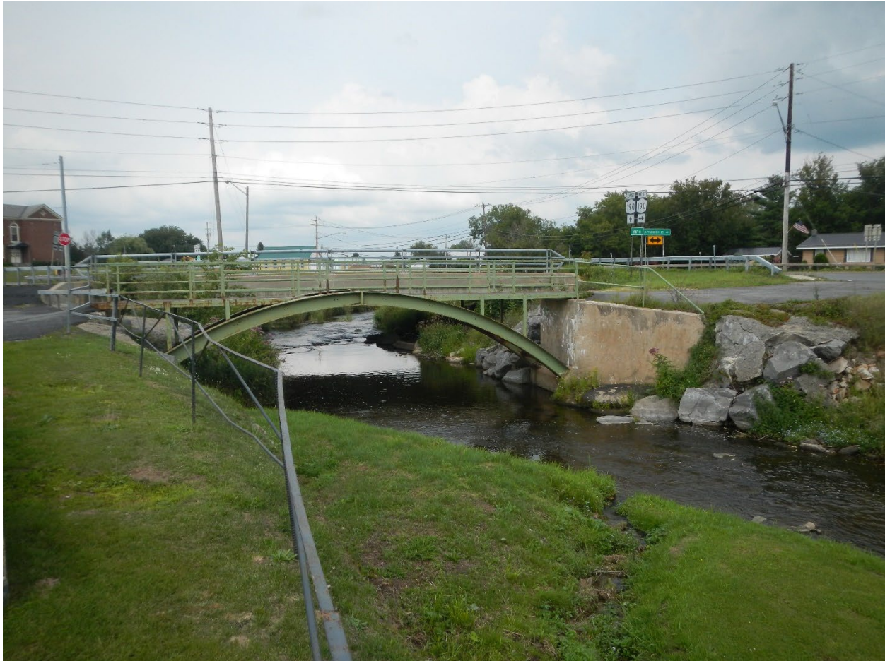
Figure 4-58: Steel Arch Pedestrian Bridge with NY-11/Military Turnpike Intersection Bridge in Background
