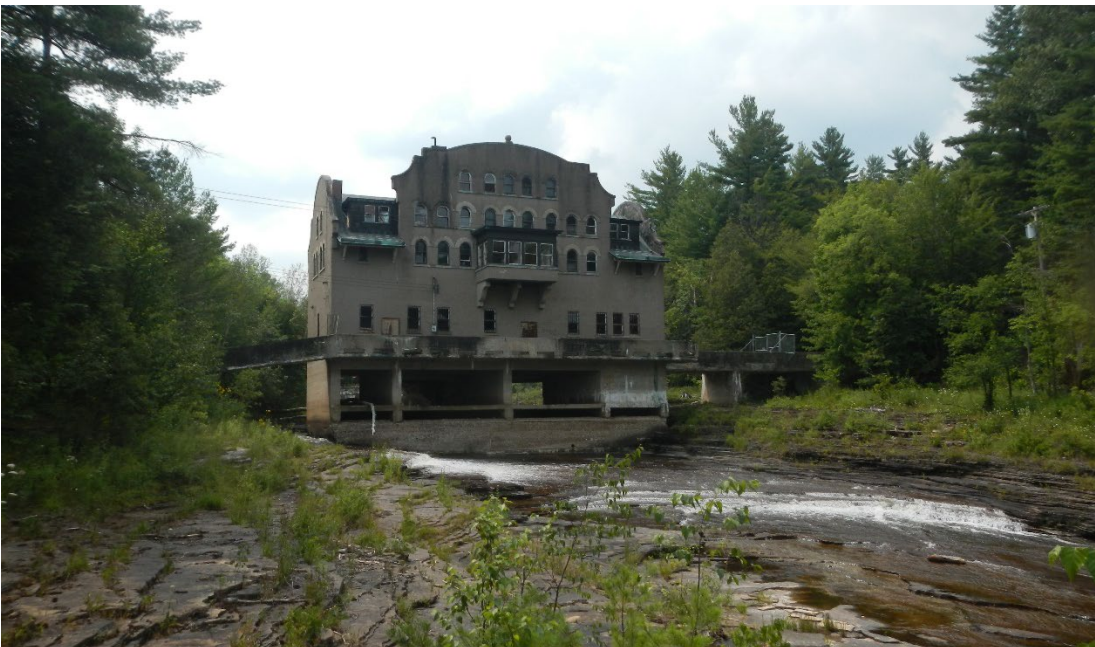
Figure 4-53: McGregor Powerhouse, constructed across the Great Chazy River. Normal flows pass around the right side of the building (left side in image).
