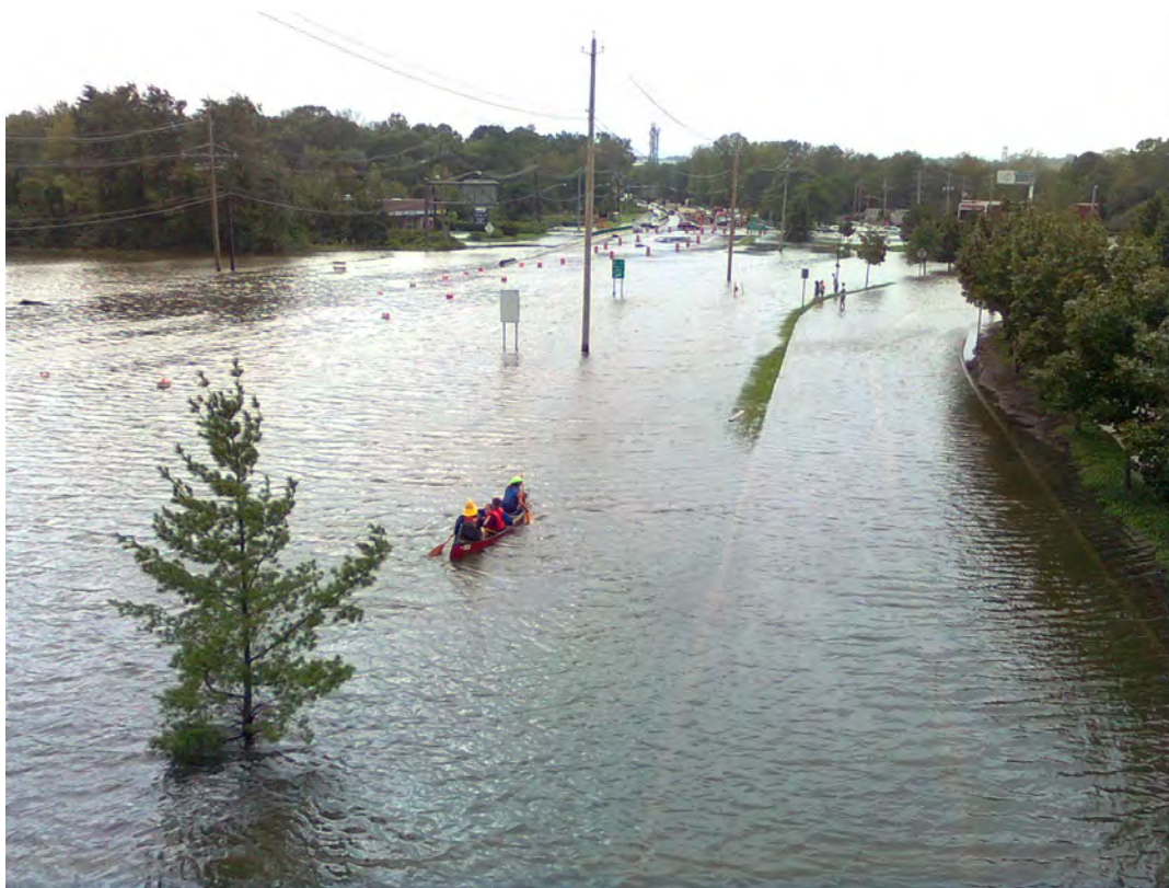
Figure 4-4: Portion of NYS Route 59 near Palisades Center Drive Under Water during Tropical Storm Irene in 2011
