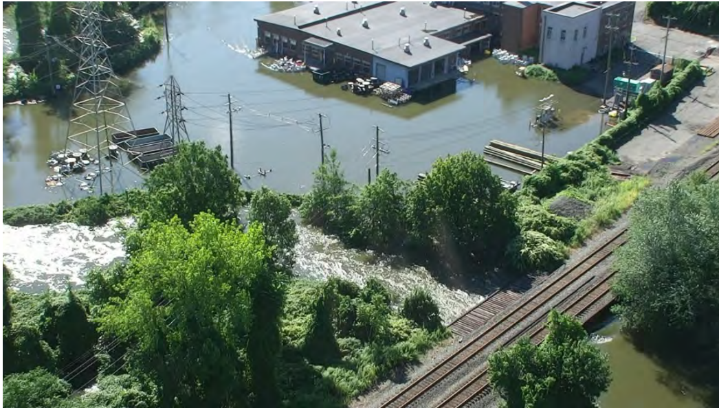
Figure 4-3: Flooding behind the Con Edison West Nyack Electric Utility Company Facility during September 2021 flood. CSX Bridge #2 at STA 294+50 is at bottom-right.
