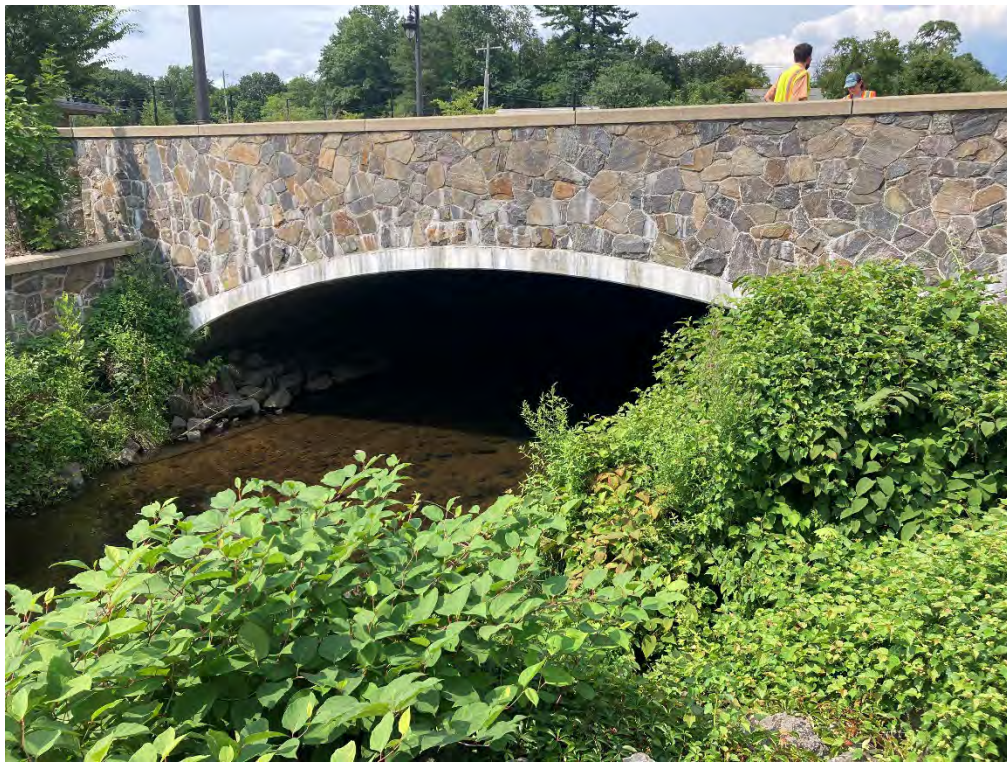
Figure 4-28: Recently Replaced New Hempstead Road Bridge
