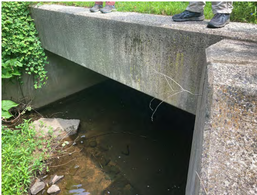
Figure 4-31: Blauvelt Road Box Culvert
