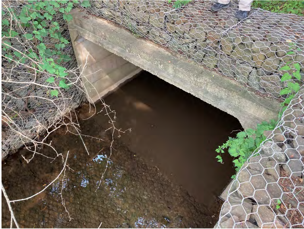
Figure 4-15: One of the Twin Box Culverts Under Squadron Drive
