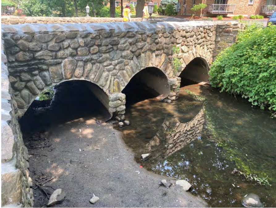
Figure 4-42: One of the Triple-Pipe Arch Culvert Bridges in Normandy Village
