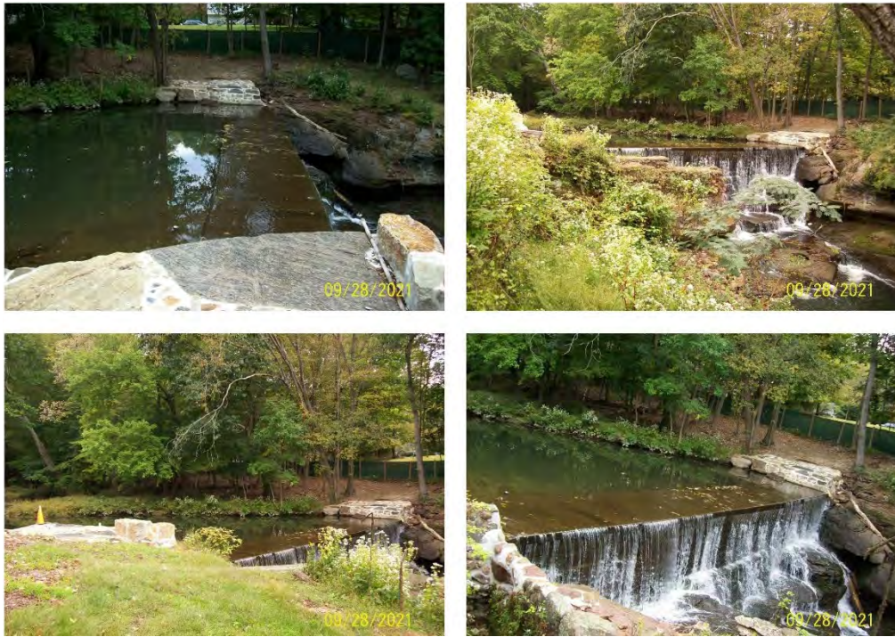
Figure 4-74: Mill Dam on Pascack Brook (photos provided by Rockland Drainage Authority)
