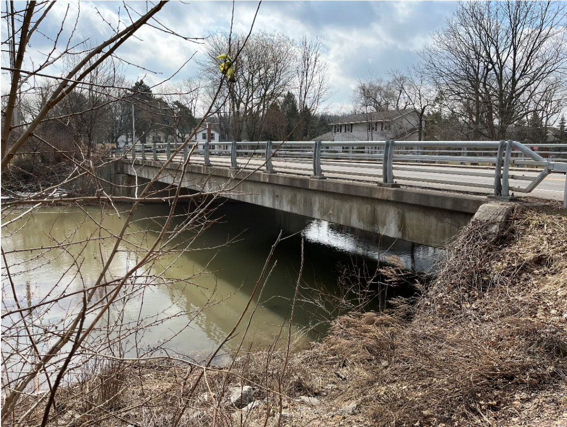
Figure 7-19. Ontario Street/NY-65 bridge, Honeoye Falls, NY.
