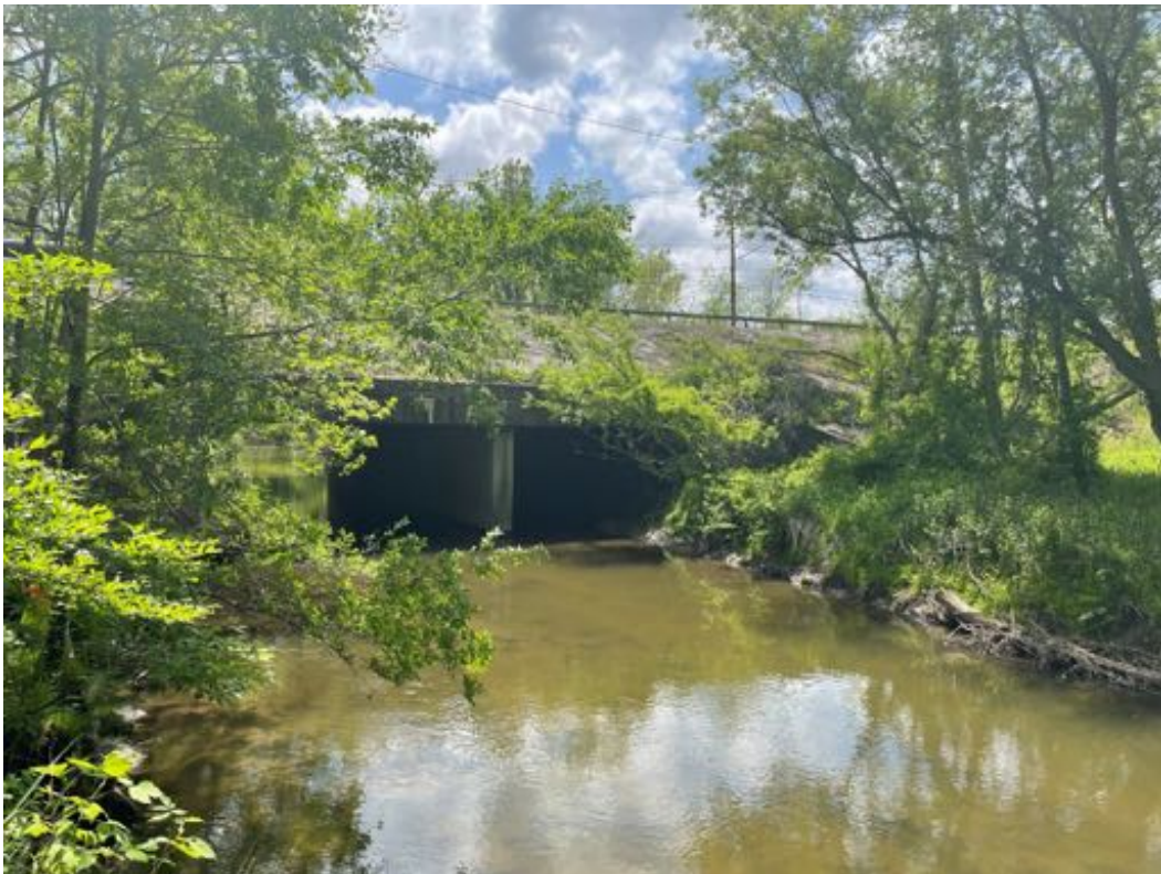
Photo D-6. Downstream Face of NY 31 (Pittsford Palmyra Road)
