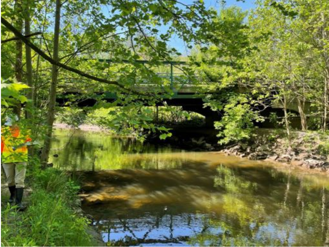
Photo D-1. Downstream Face of Old Penfield Road
