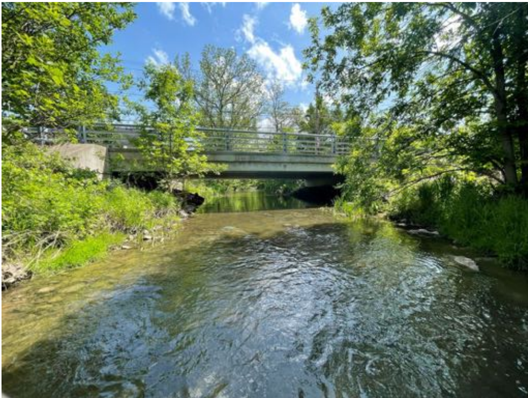
Photo D-8. Downstream Face of NY 251 (Victor Mendon Road)
