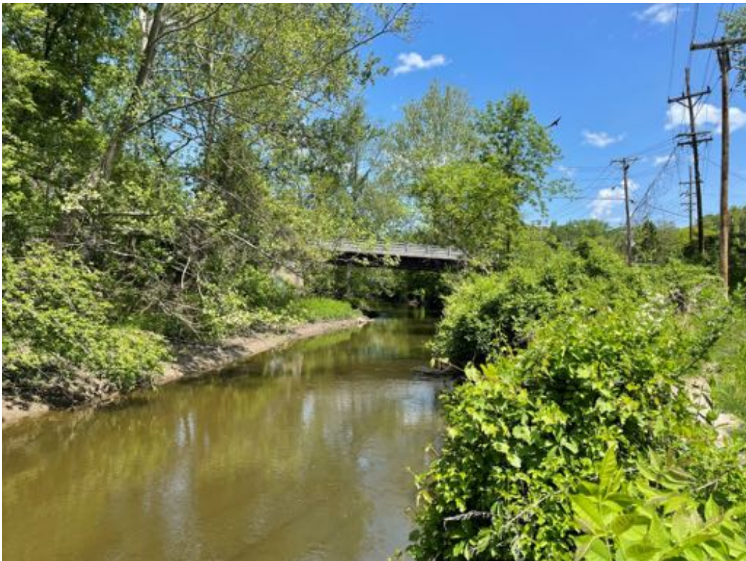
Photo D-2. Upstream Face of Penfield Road
