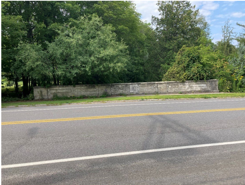
Figure 4-21: West Church Street bridge, looking downstream across the road surface
