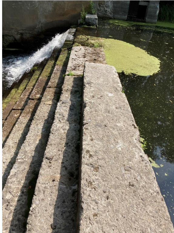
Figure 4-7: Spillway of the W.H. Miner Dam #2 in West Chazy
