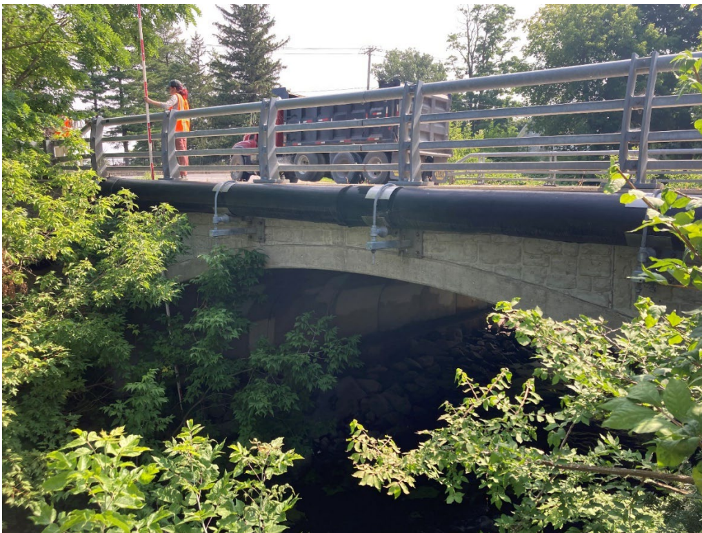
Figure 4-13: Fiske Road concrete arch bridge, looking upstream from the left bank
