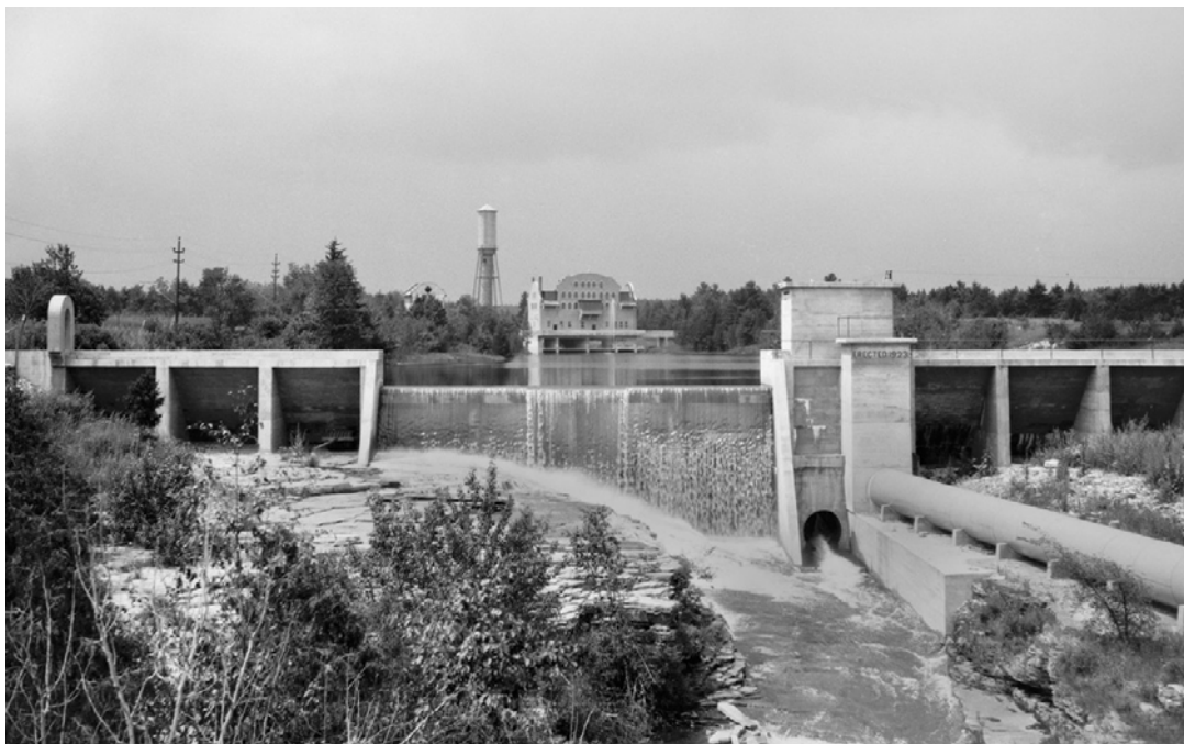
Figure 4-33: LaSell Dam on the Great Chazy River in the 1920s. McGregor Powerhouse in background.
