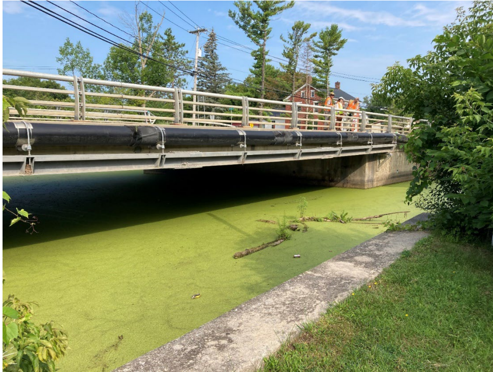
Figure 4-5: US-9 bridge, right training wall of Little Chazy Dam in foreground
