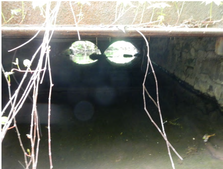
Figure 4-29 Inlet Pipes on Culvert at Viola Road Crossing Viewed from Outlet
