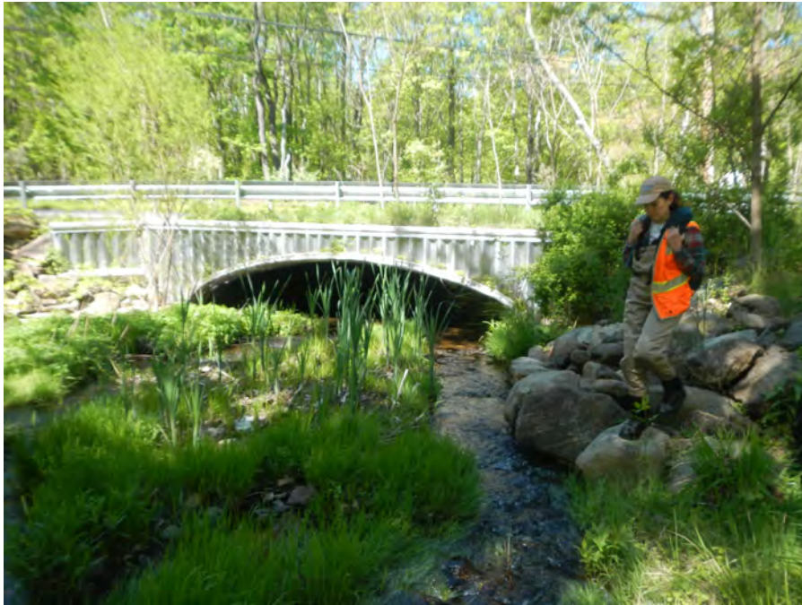
Figure 4-34 Mountain Road Crossing over Mahwah River
