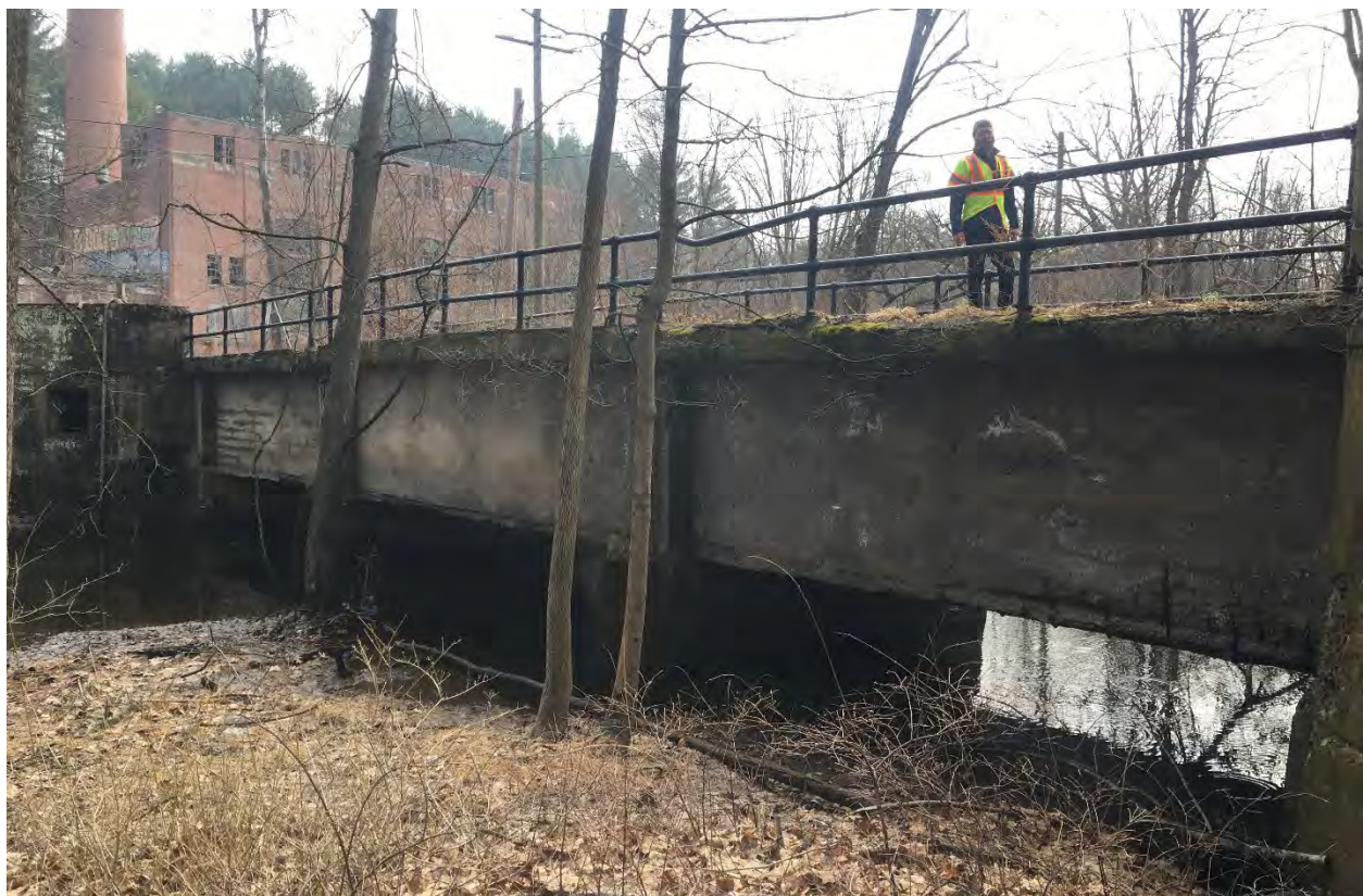
Figure 4-23: Rockland Print Company Power Plant Bridge
