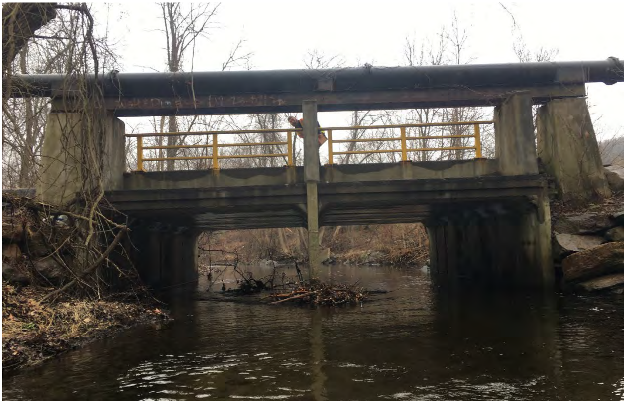
Figure 4-24: West Haverstraw DPW Facility Bridge
