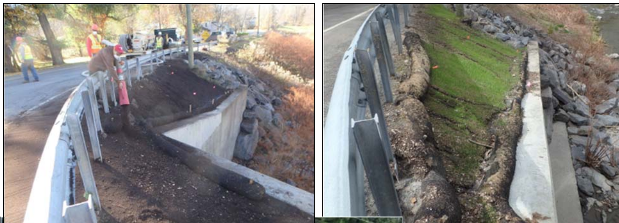
Before and after photos of compost socks installed in November 2016 on a slope above waterway in Brooktondale, NY. The socks prevented erosion and reduced roadside pollutants from reaching surface water by acting as a filter
