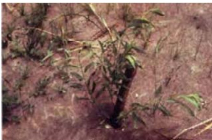
Shown above: A live stake installed to create a living root mat that stabilizes the soil after construction along a raw streambank. Live stakes are one of the many erosion and sediment control techniques found in the New York State Standards and Specifications for Erosion and Sediment Control (shown right).
